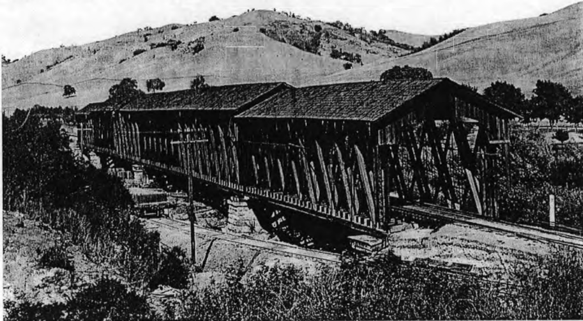
Covered Howe truss bridge at Arroyo de la Laguna (Sunōl Creek) just before replacement. Note temporary bypass track in foreground.
