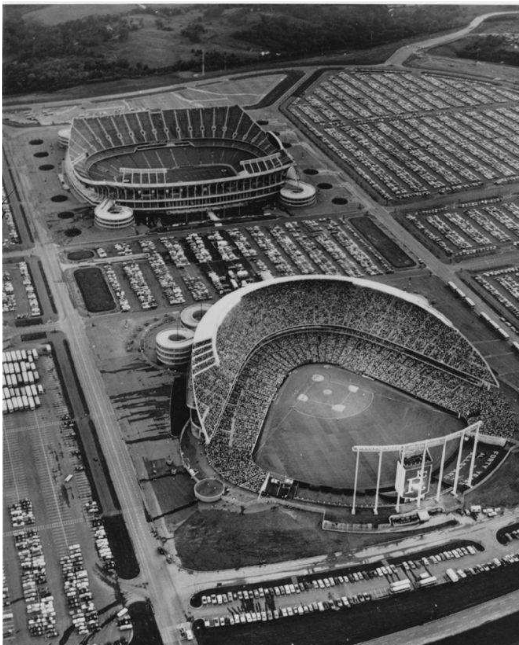
Figure 22: Truman Sports Complex, date unknown. (Source: Missouri Valley Special Collections, Kansas City Public Library, accessed online 31 March 2015).
