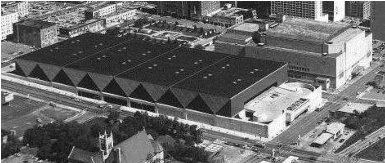
Figure 23: Bartle Hall Convention Center, Kansas City, c. mid-1970s (Source: Robert Askren Photograph Collection, Missouri Valley Special Collections, Kansas City Public Library, accessed online 30 October 2013).
