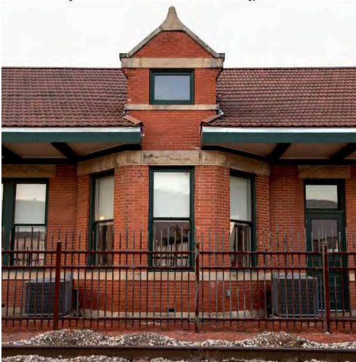
Photo 2: Bay window detail—camera facing north
