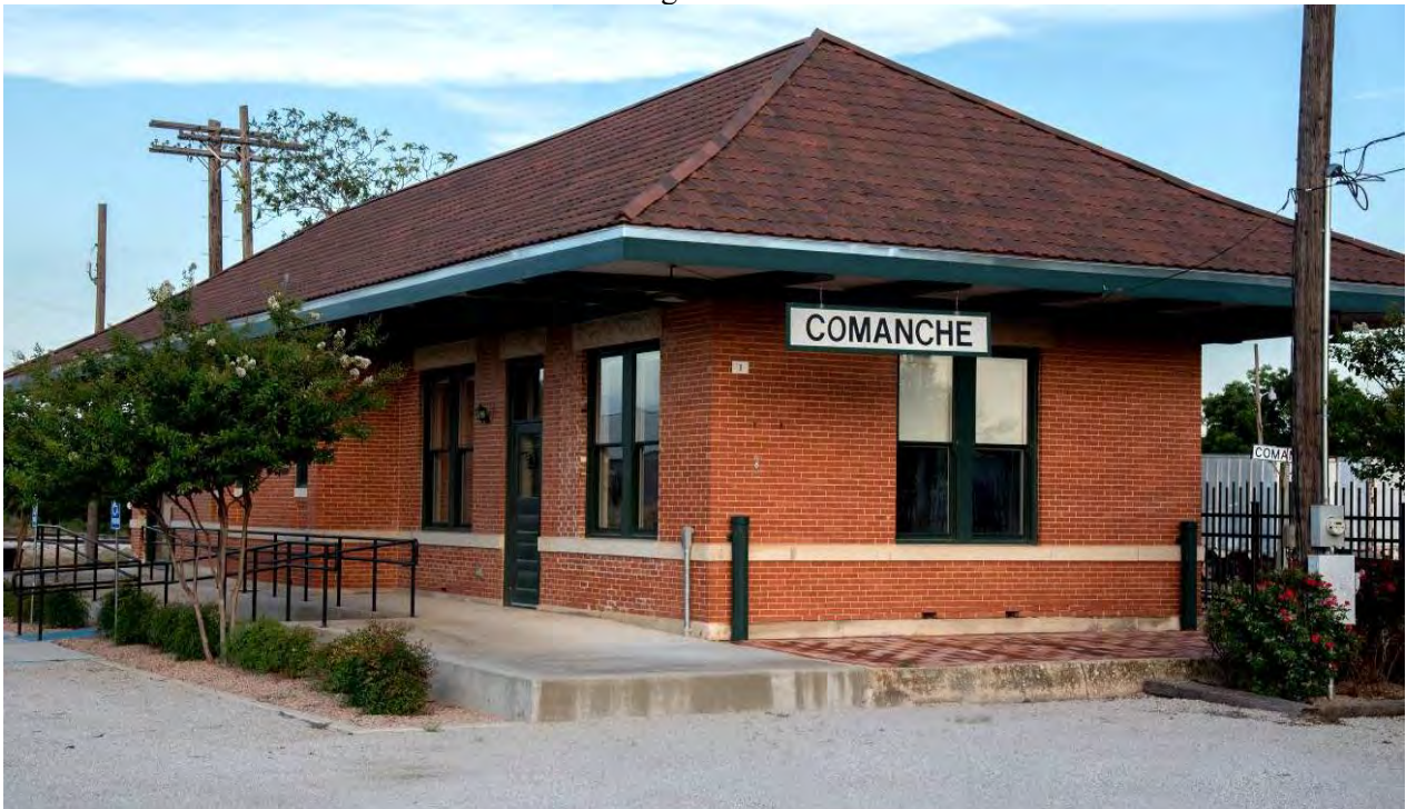
Photo 6: North and west elevations—camera facing southeast
