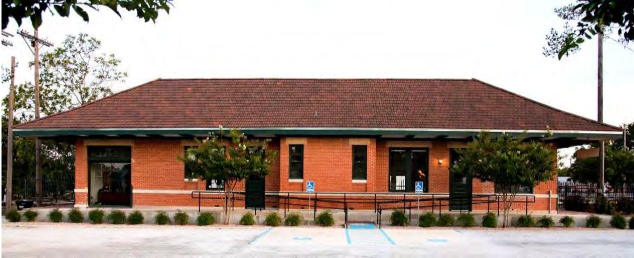
Photo 5: North elevation—camera facing south
