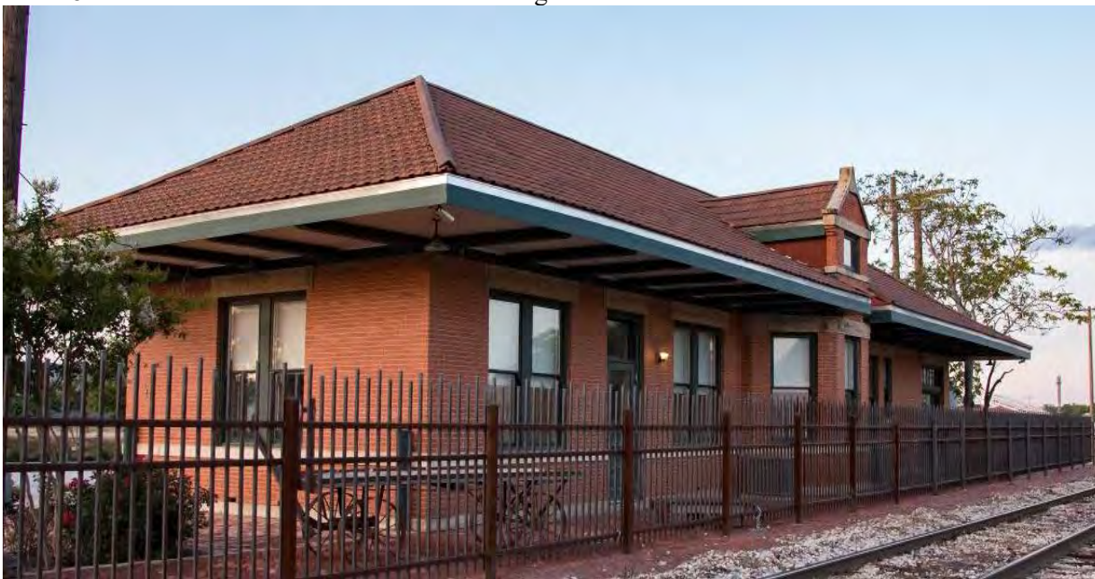
Photo 8: South and west elevations—camera facing northeast
