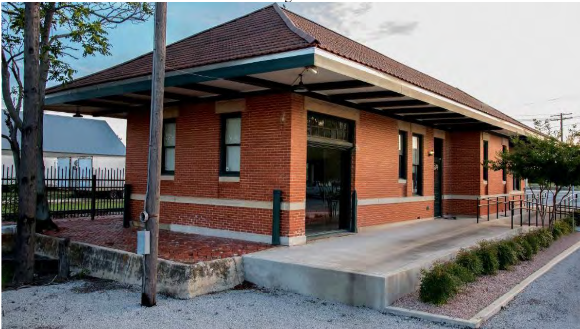
Photo 4: North and east elevations—camera facing southwest
