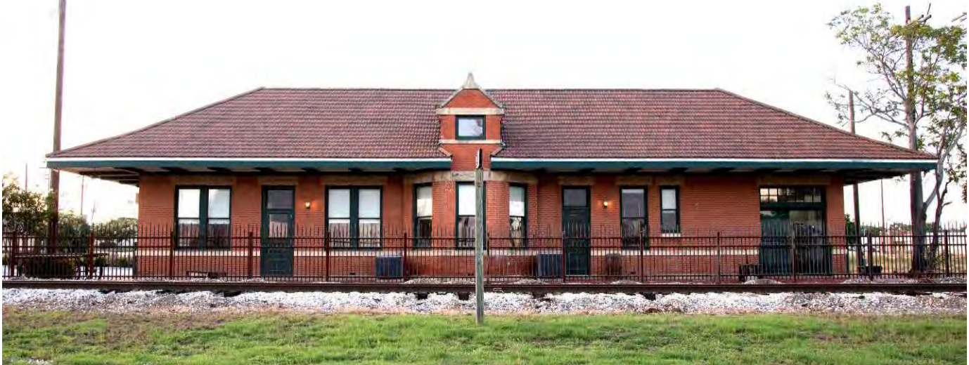
Photo 1: South elevation—camera facing north
