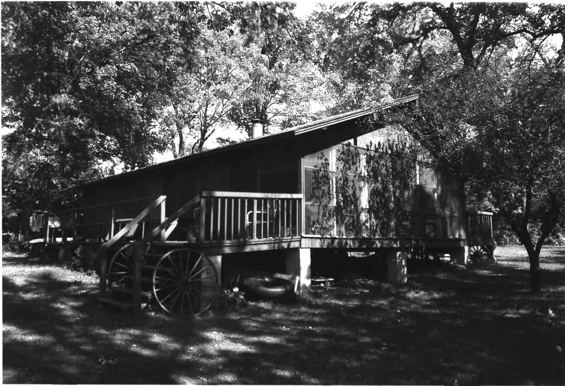
LOT 21, CRANE ISLAND HISTORIC DISTRICT HENNEPIN CO., MN. PHOTO I.D. # 010863 - 8A/9 NON-CONTRIBUTING
