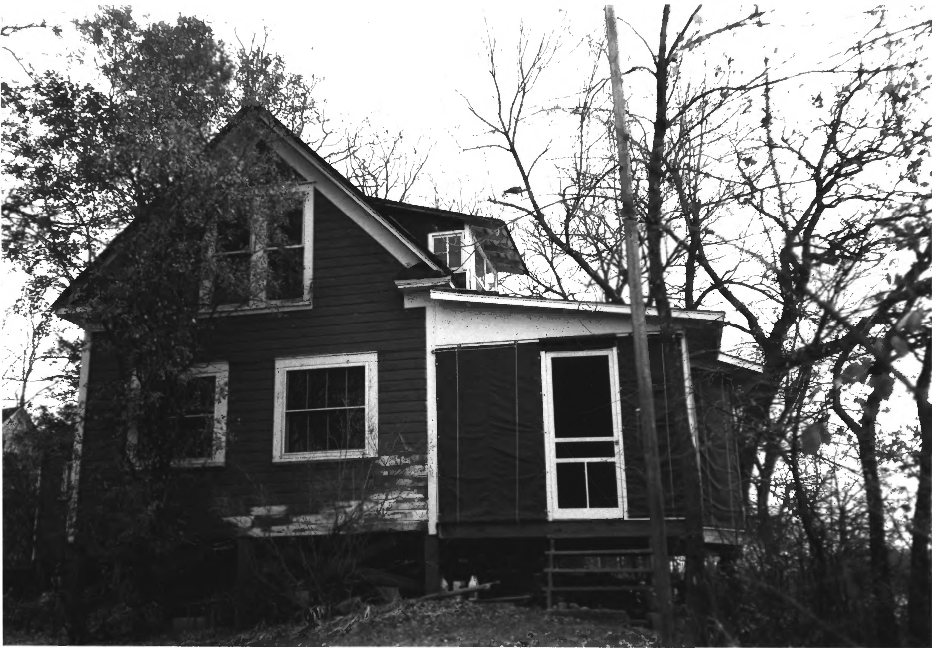
LOT 3, CRANE ISLAND HISTORIC DISTRICT HENNEPIN CO., MN PHOTO I.D. # 010864 - 3/3A
