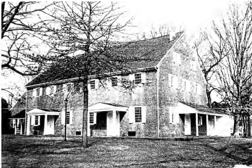
Figure 20: Union Street or Upper Evesham (Orthodox) Friends Meeting House, Medford, NJ, built in 1814.
