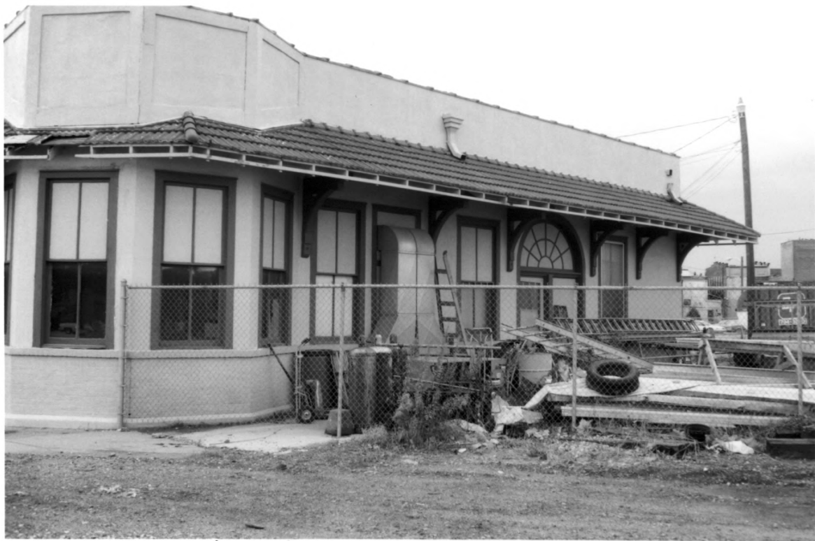
Union City Mobile and Ohio Railroad Depot #7df22 Obion Co. TN
