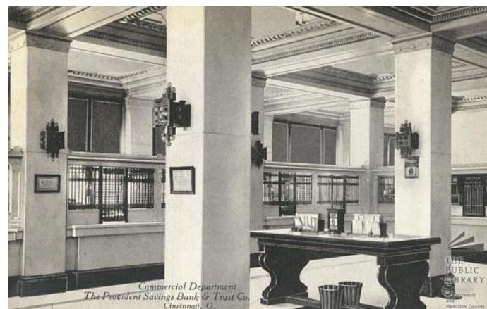
Banking hall interior, 1908
