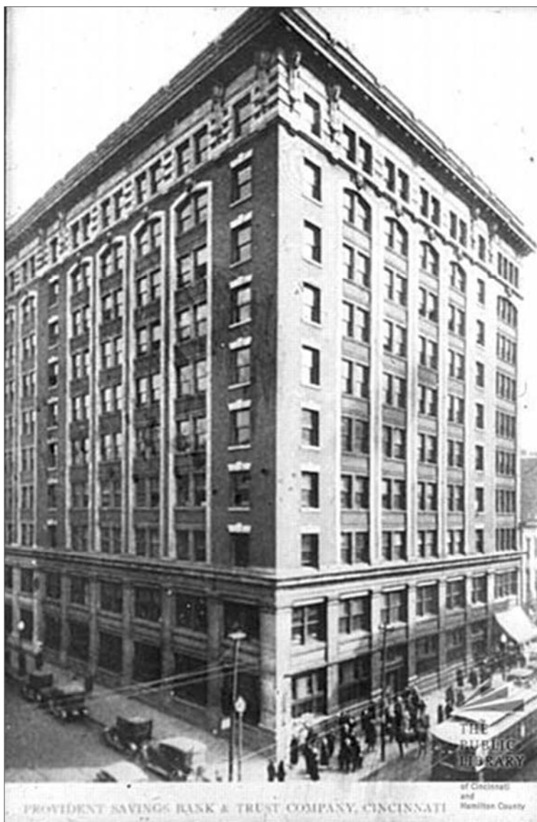
After both additions added, post 1923
