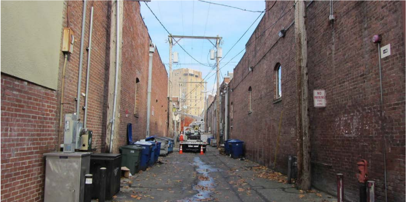
7 of 18. Typical alley view from West Holly Street looking northeast.
