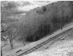
Figure 22: View of the railroad line as it begins to make its curve to the southeast.
