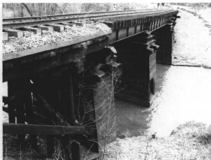
Figure 2: Big Lost Creek Bridge just west of Probst .
