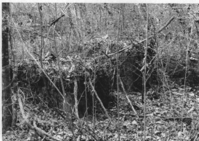
Figure 19: House foundations at Apalachia.
