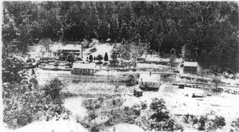
Figure 32: McFarland, ca. 1920, showing the two-story hotel and dwellings (Alice Presswood collection: Photo courtesy of the Polk County News).
