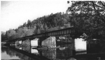
Figure 1: Knoxville Southern Railroad Bridge over the Hiwassee River at Reliance.
