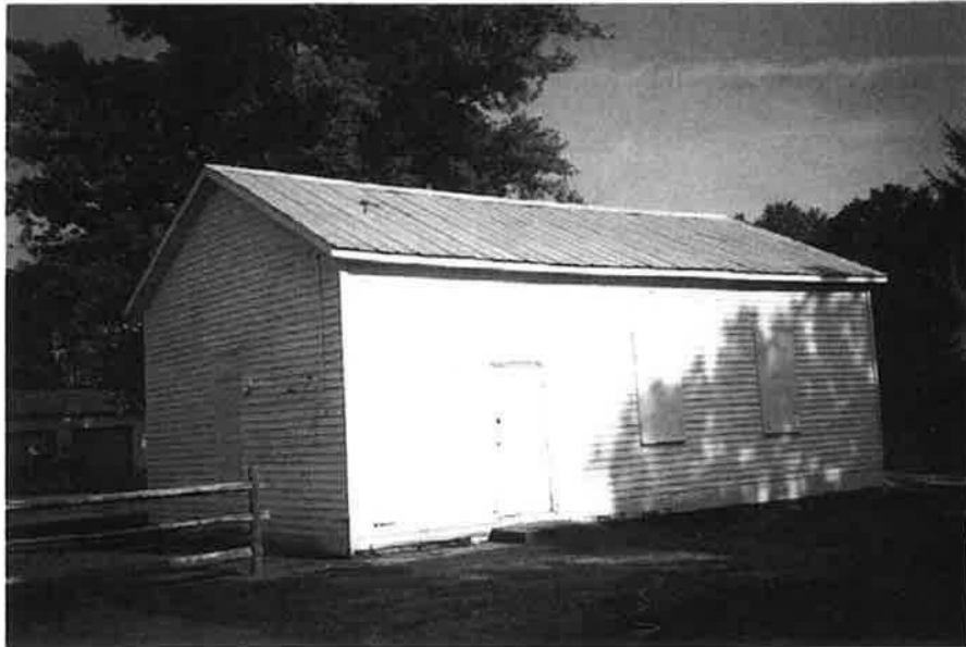
Morgan Township House, ca. 2001. South and East Elevations.
