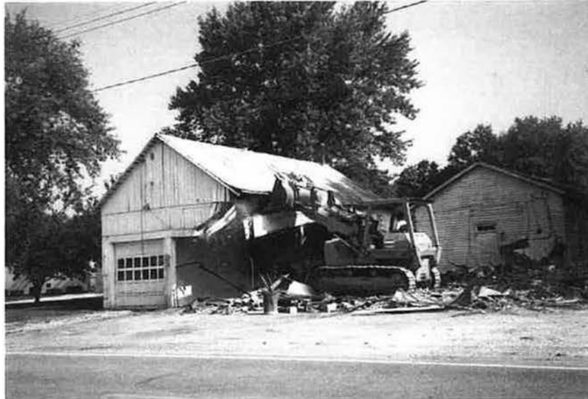
Morgan Township House. Site Demolition. August 29, 2000.
