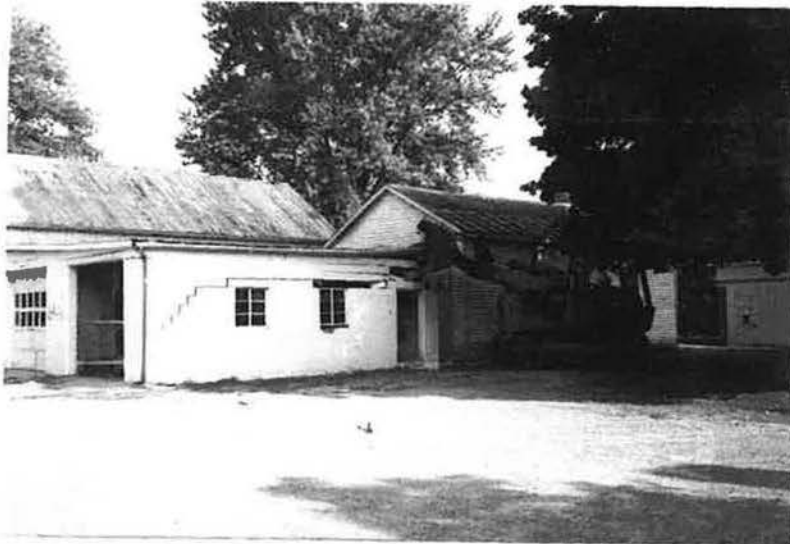
Morgan Township House Additions. Site Demolition. August 2000.
