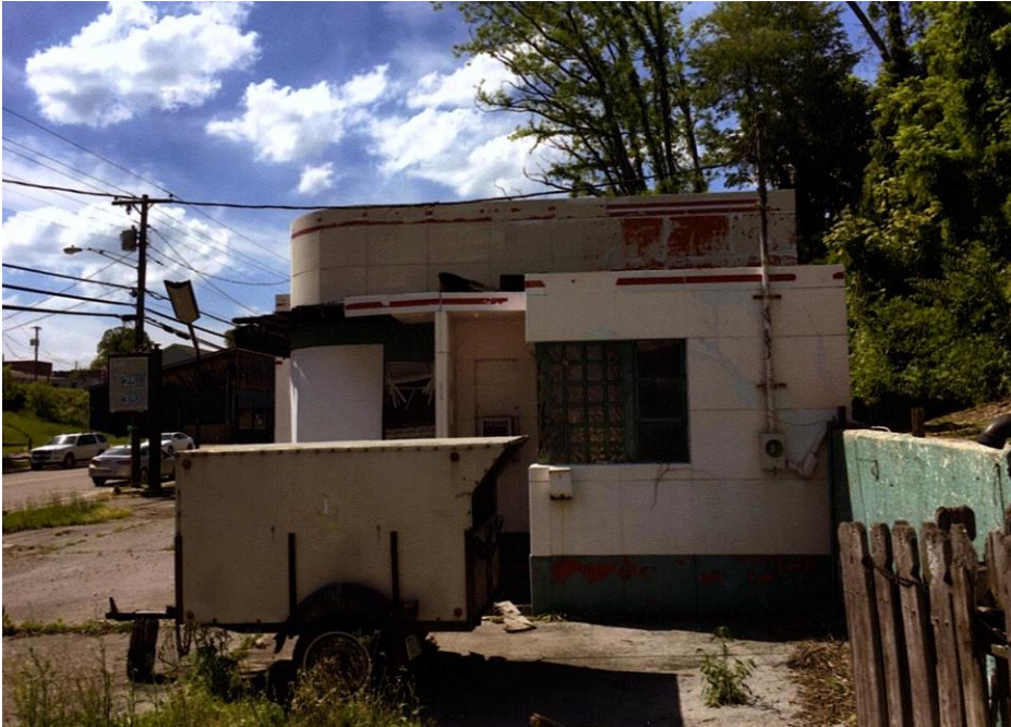
Photo 5: East elevation, facing west
