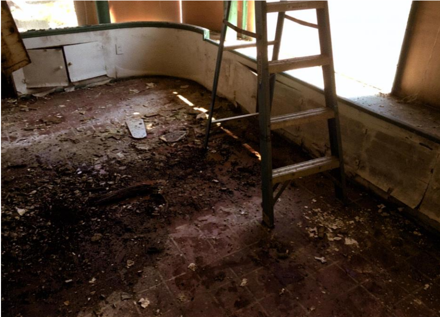
Photo 10: Interior, view of east elevation and south elevation (façade), facing southeast
