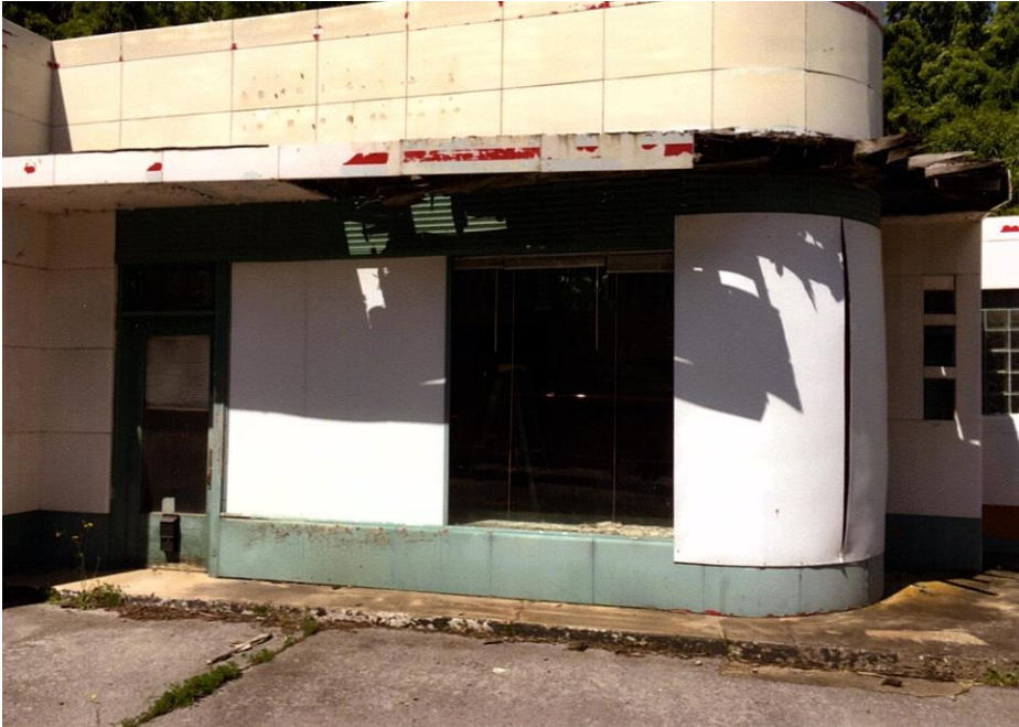
Photo 3: Exterior view of office area/display windows, facing north
