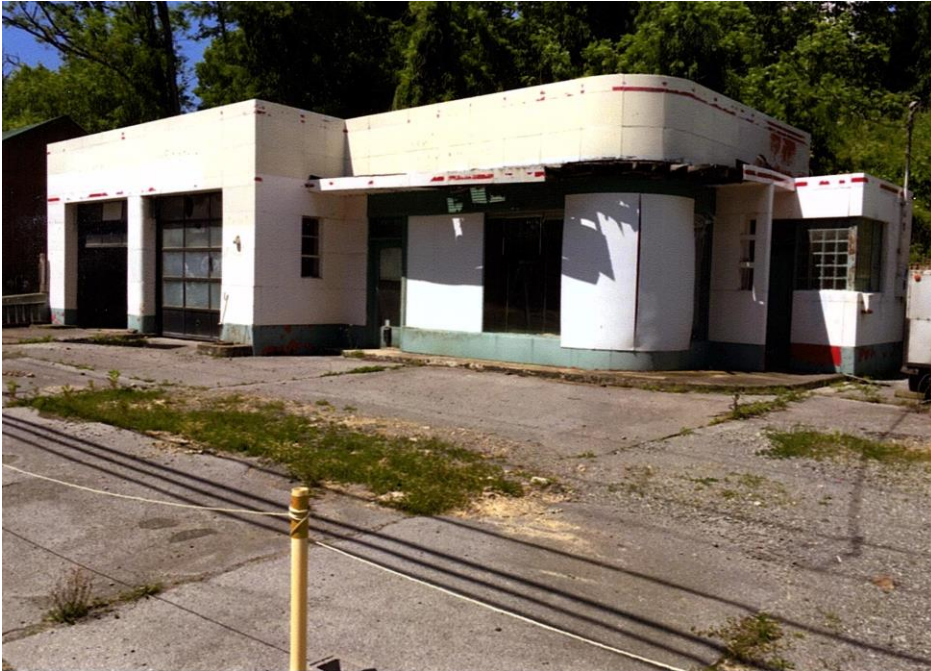
Photo 1: Southeast Elevation, facing NW
