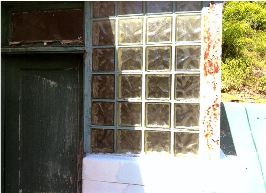
Photo 6: East Elevation, Glass block partition, facing north
