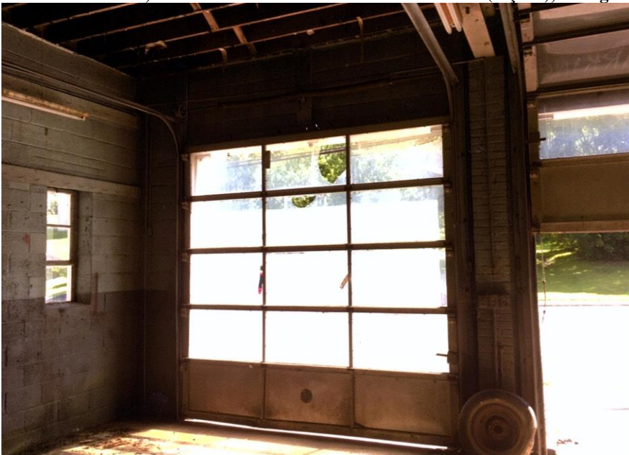
Photo 11: Interior, view of eastern most service bay, facing south
