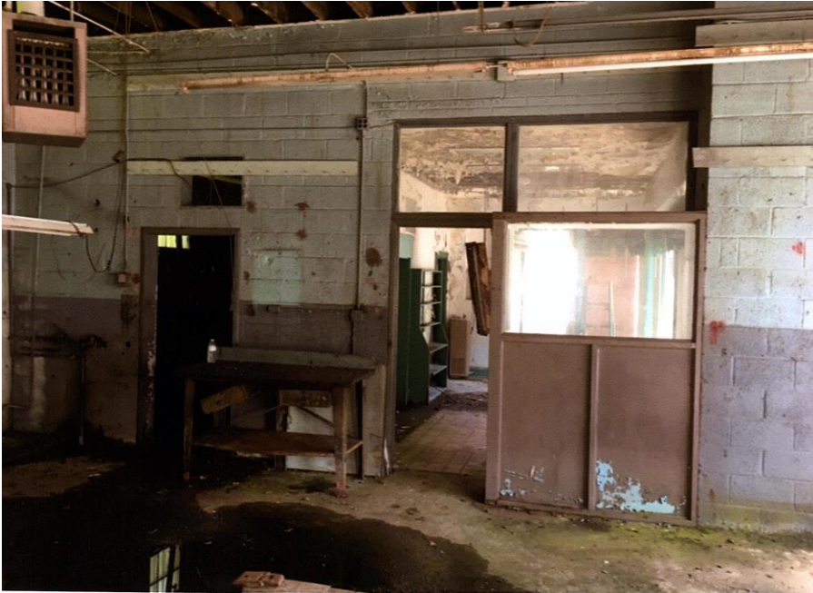
Photo 7: Interior, east service bay, facing east (toward office area)
