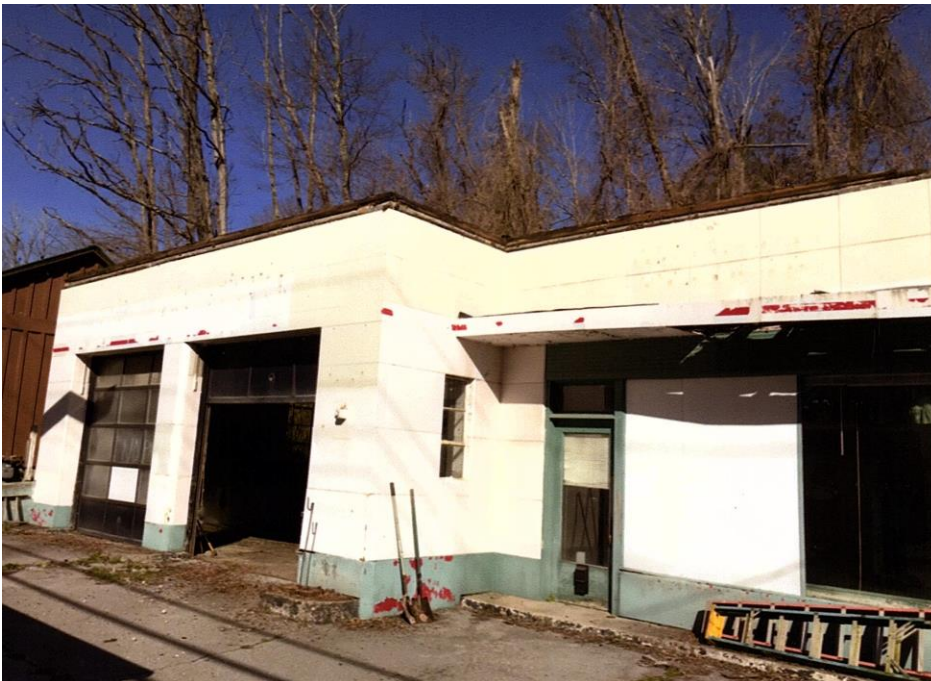
Photo 2: Façade (south elevation), garage doors to the north, facing NW
