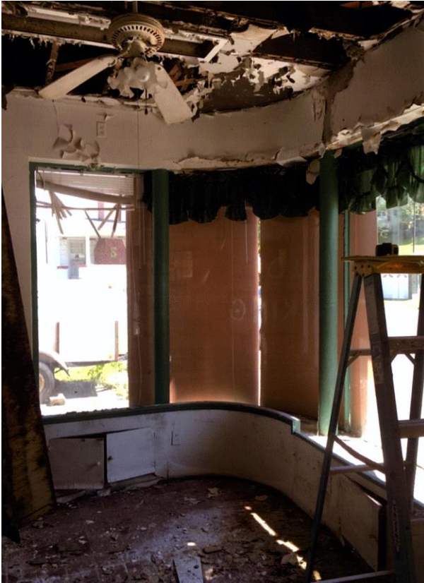
Photo 9: Interior, office area, curved south facing glass and wall, facing southeast
