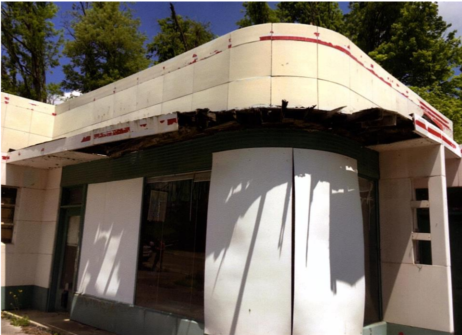
Photo 4: South facade and east elevation (partial), facing NW
