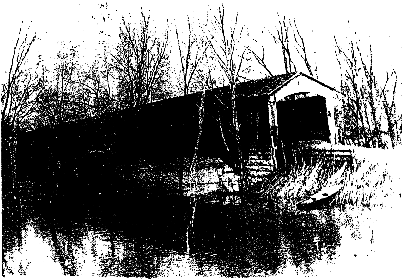
BRIDGE IN MEDORA JULY 19 1913
