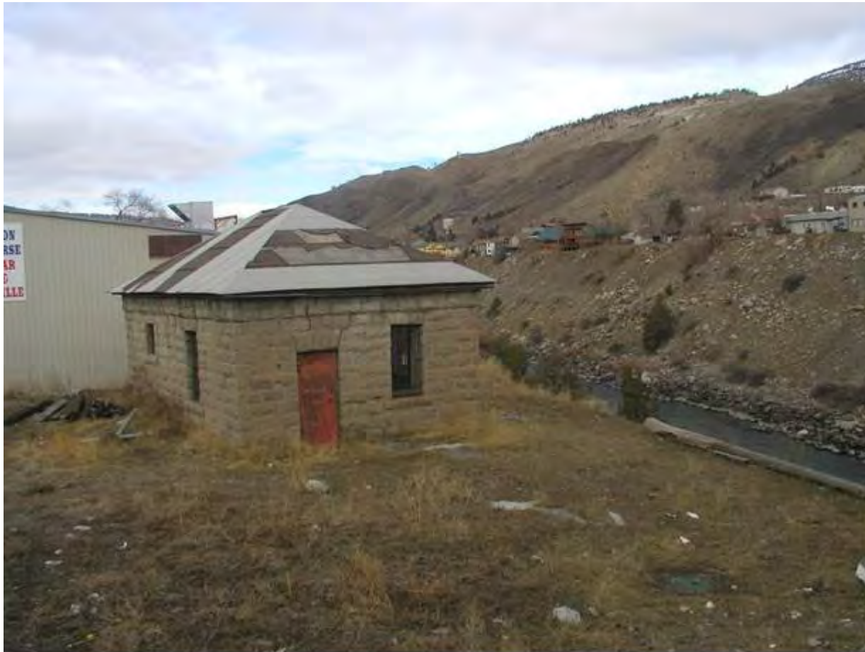
Description and view of camera: East and South elevation, view to northwest Photograph: MT_ParkCounty_GardinerJail_0003
