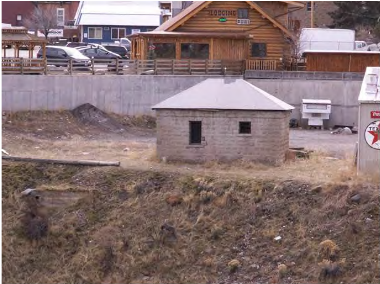
Description and view of camera: North elevation, view to south Photograph: MT_ParkCounty_GardinerJail_0006
