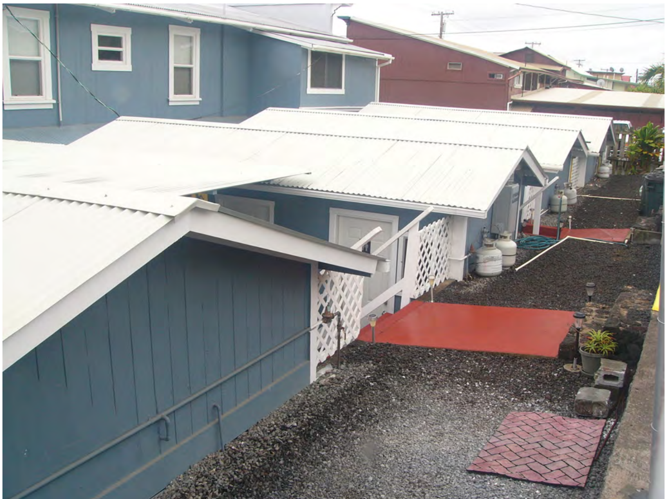
Photo #4 (HI_Hawai'iCounty_Ferreira Building_0004) Out buildings (mauka side)partial, camera facing east-southeast. Photographer: Annalise Kehler
