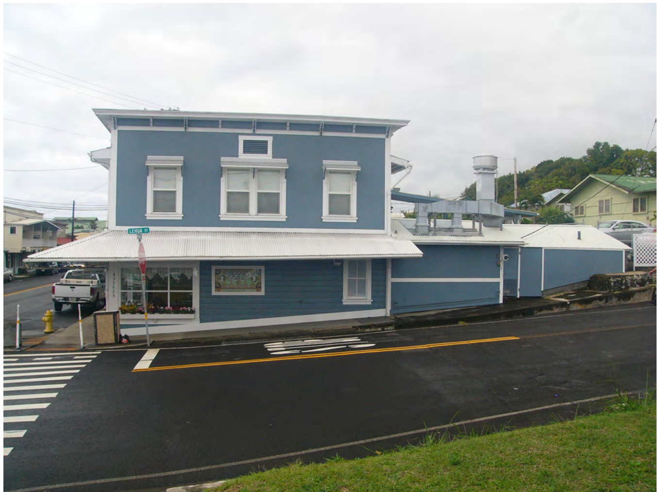
Photo #3 (HI_Hawai'iCounty_Ferreira Building_0003) Lehua Street (Waipi'o side) façade, camera facing east-southeast. Photographer: Laura Ruby
