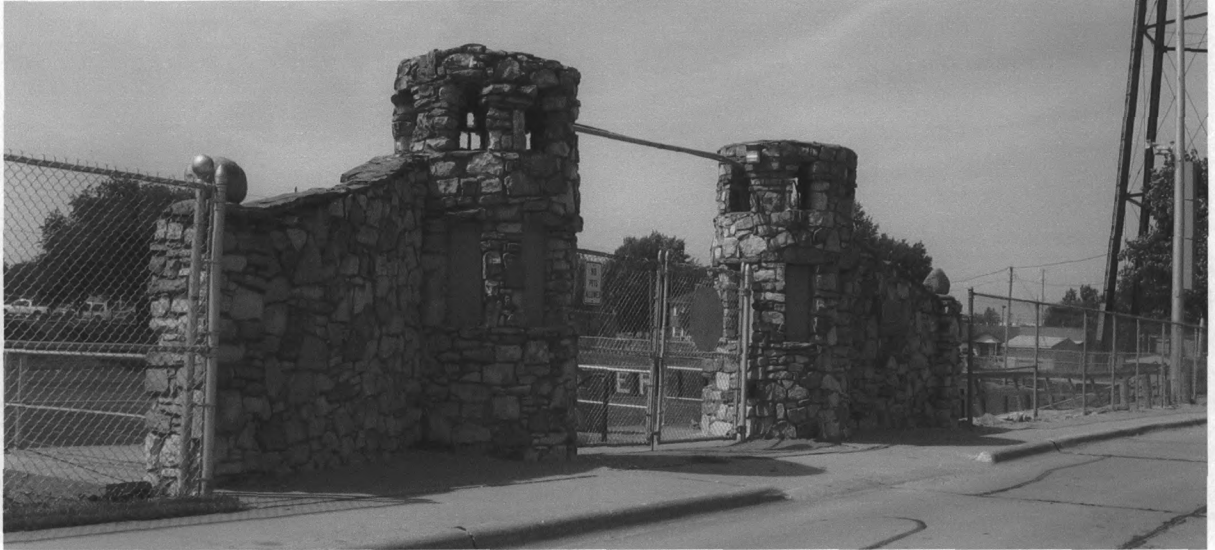
Stone gateway on east side of stadium looking NW from Stadium Street
