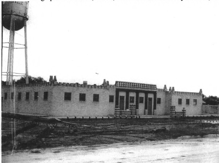
Looking SE at bath house with water tower in background, June 10, 1938
