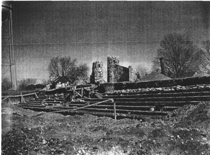
Looking NE at east side bleachers and stone gateways under construction, February 24, 1939
