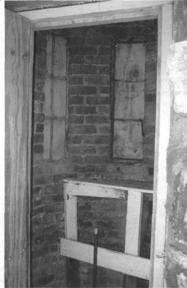
Interior of the south west-side gateway tower ticket booth
