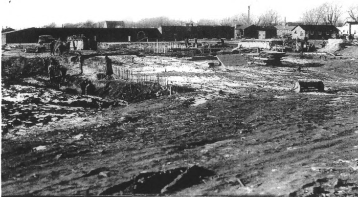
Looking NW at bath house and swimming pool excavations, December 10, 1937
