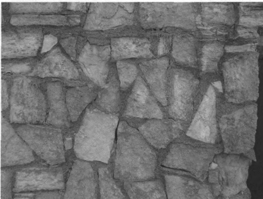
Detail of stonework in storage building
