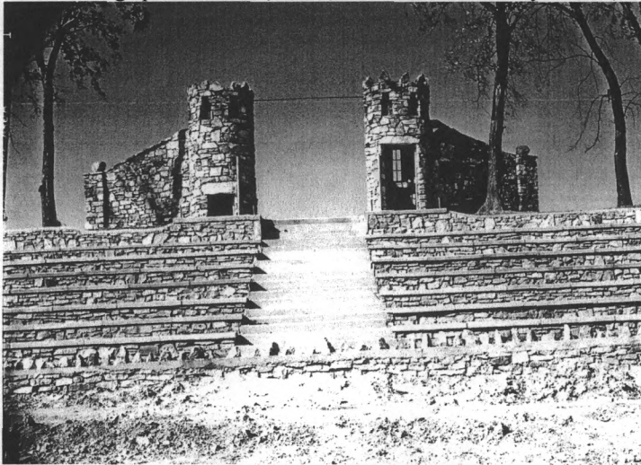
Looking West at west side stone gateway (ticket booths) and bleachers, October 14, 1938
