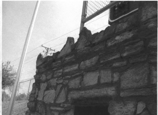
Detail of parapet stonework on storage building
