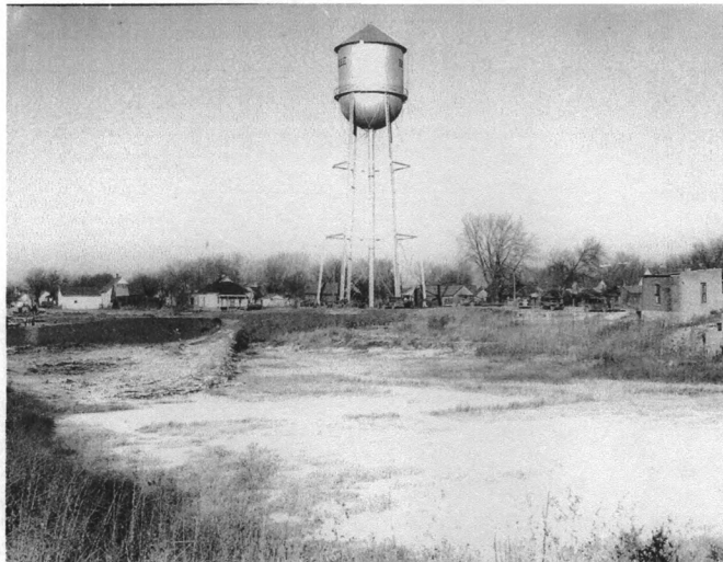
Looking to NE at WPA Pool/Athletic Field construction site and extant water tower, December 10, 1937 Source: WPA Photographs Collection, Box 8, State Historical Society of Iowa, Iowa City
