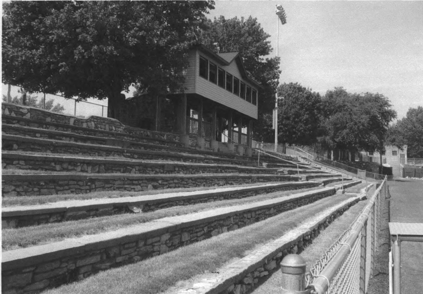
West-side bleachers and press box looking to NNW
