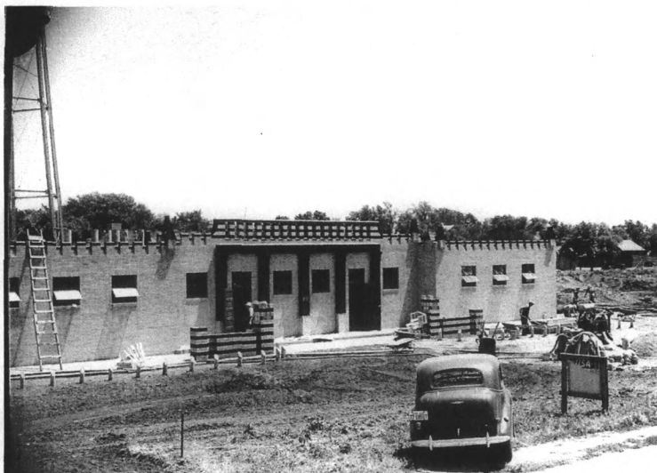
Looking ESE at bath house with water tower in background, July 1, 1938
