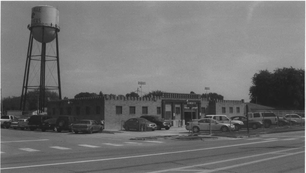
WPA Pool Bath House in foreground, looking to the ESE with water tower to left
