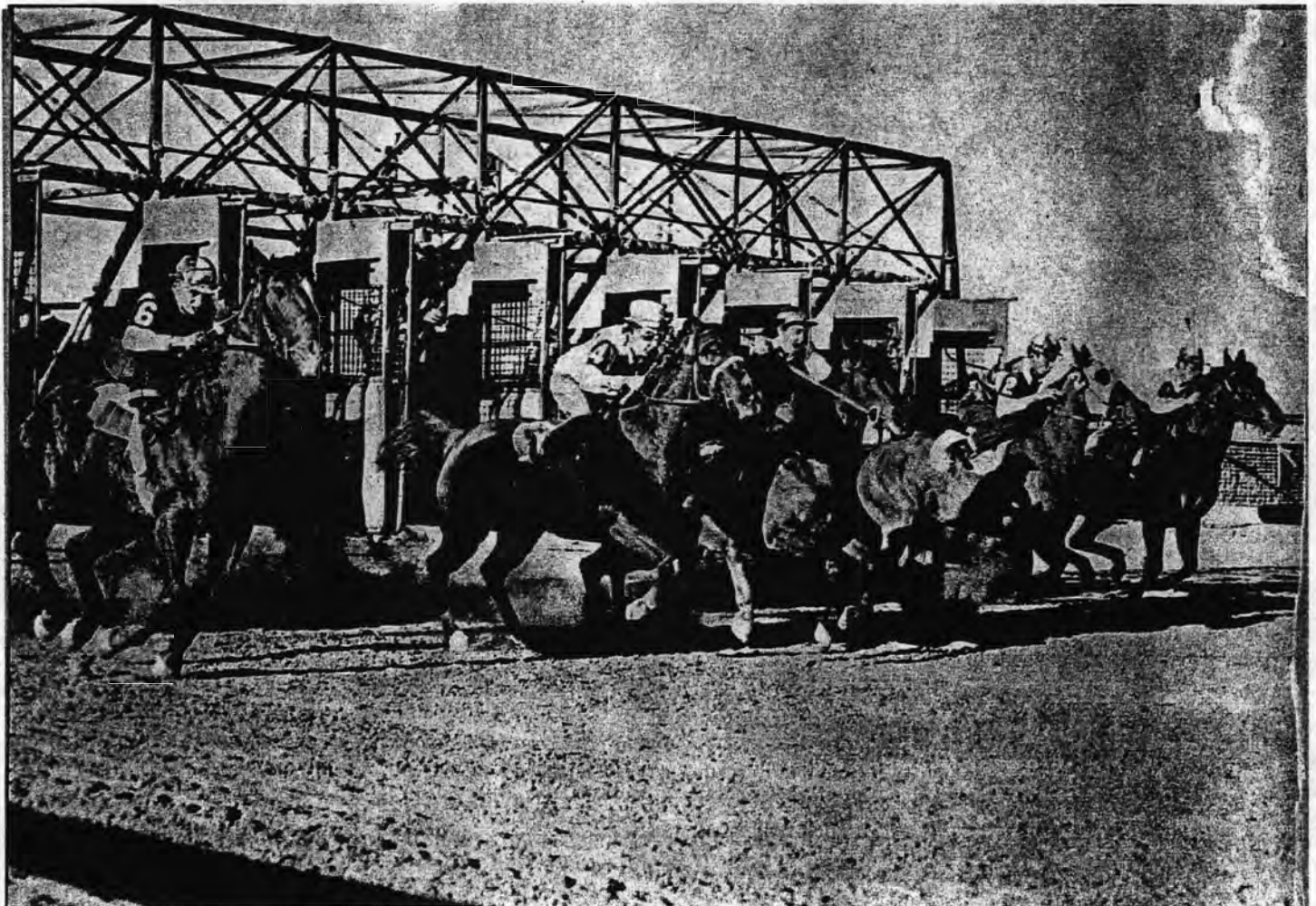
Rillito Race Track Chute, circa 1945 (Source: Jelks Archive, Race Track Industry Program, The University of Arizona)
