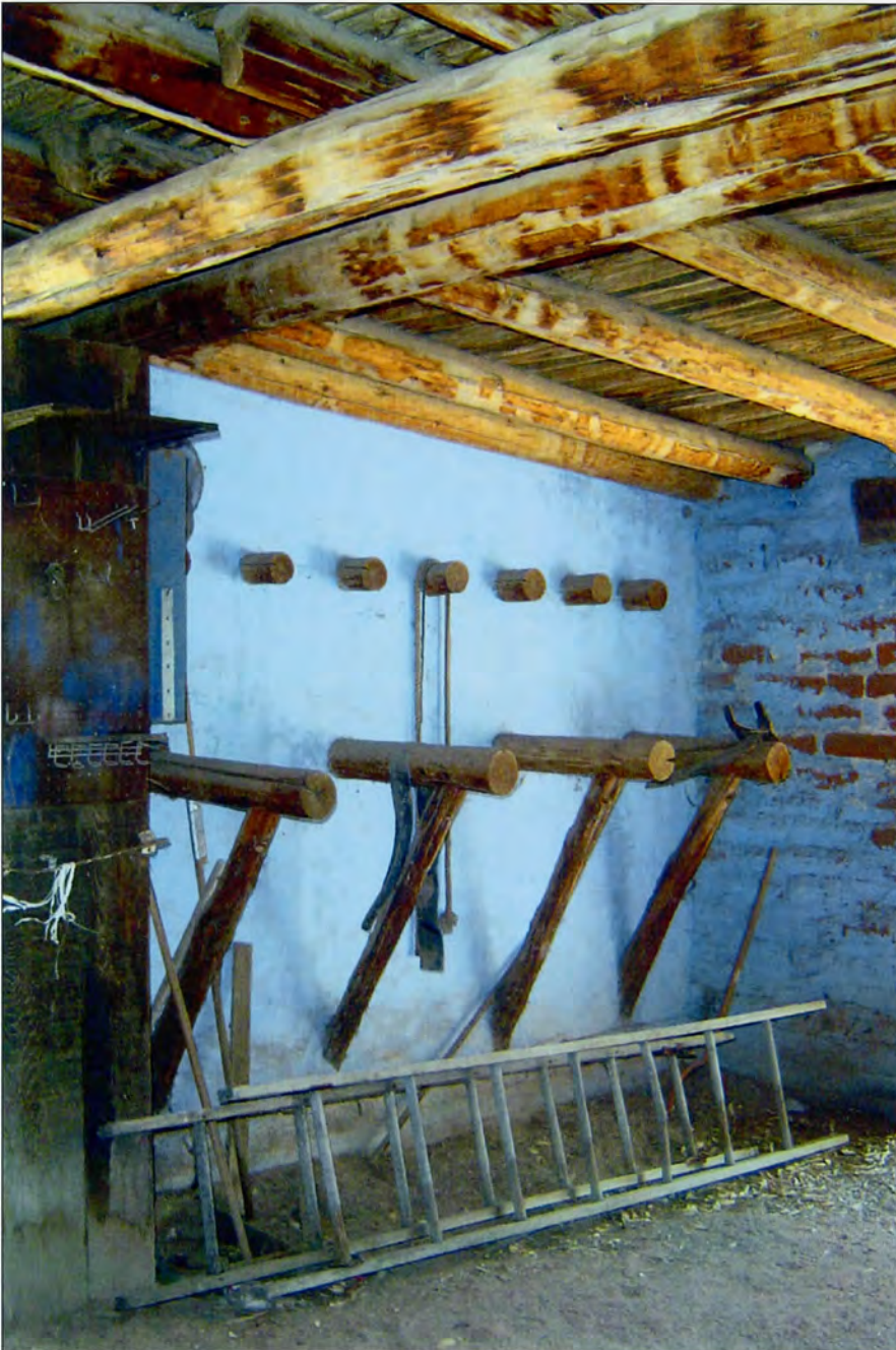
PHOTO #18: Interior view of the stables tack area facing southeast, 4/2008
