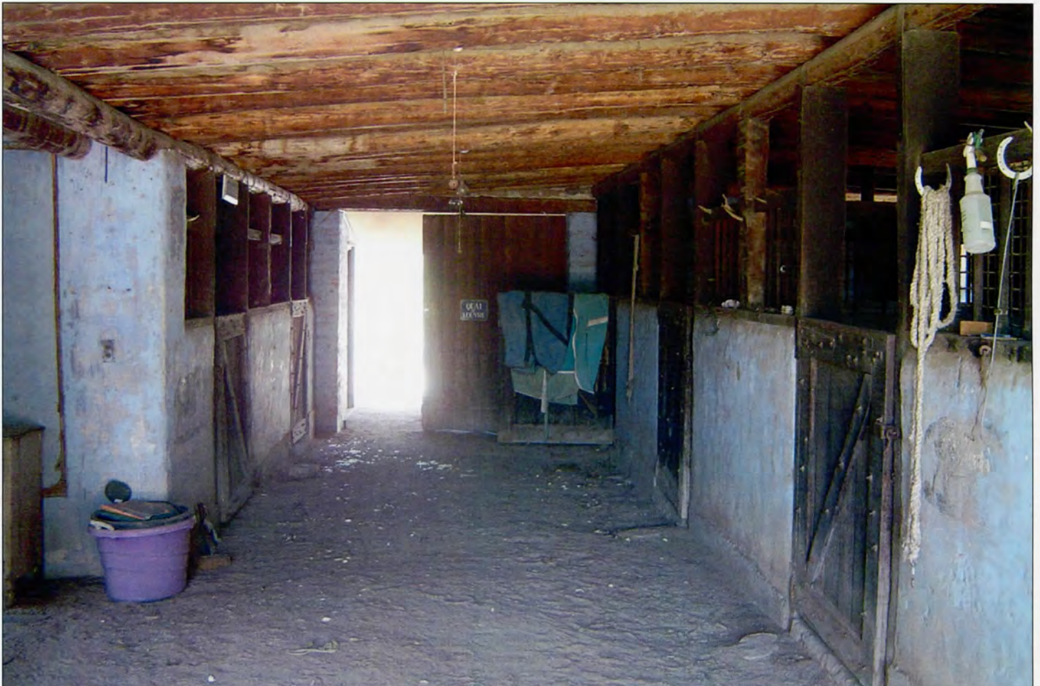
PHOTO #17: Interior view of the stables corridor facing west, 4/2008
