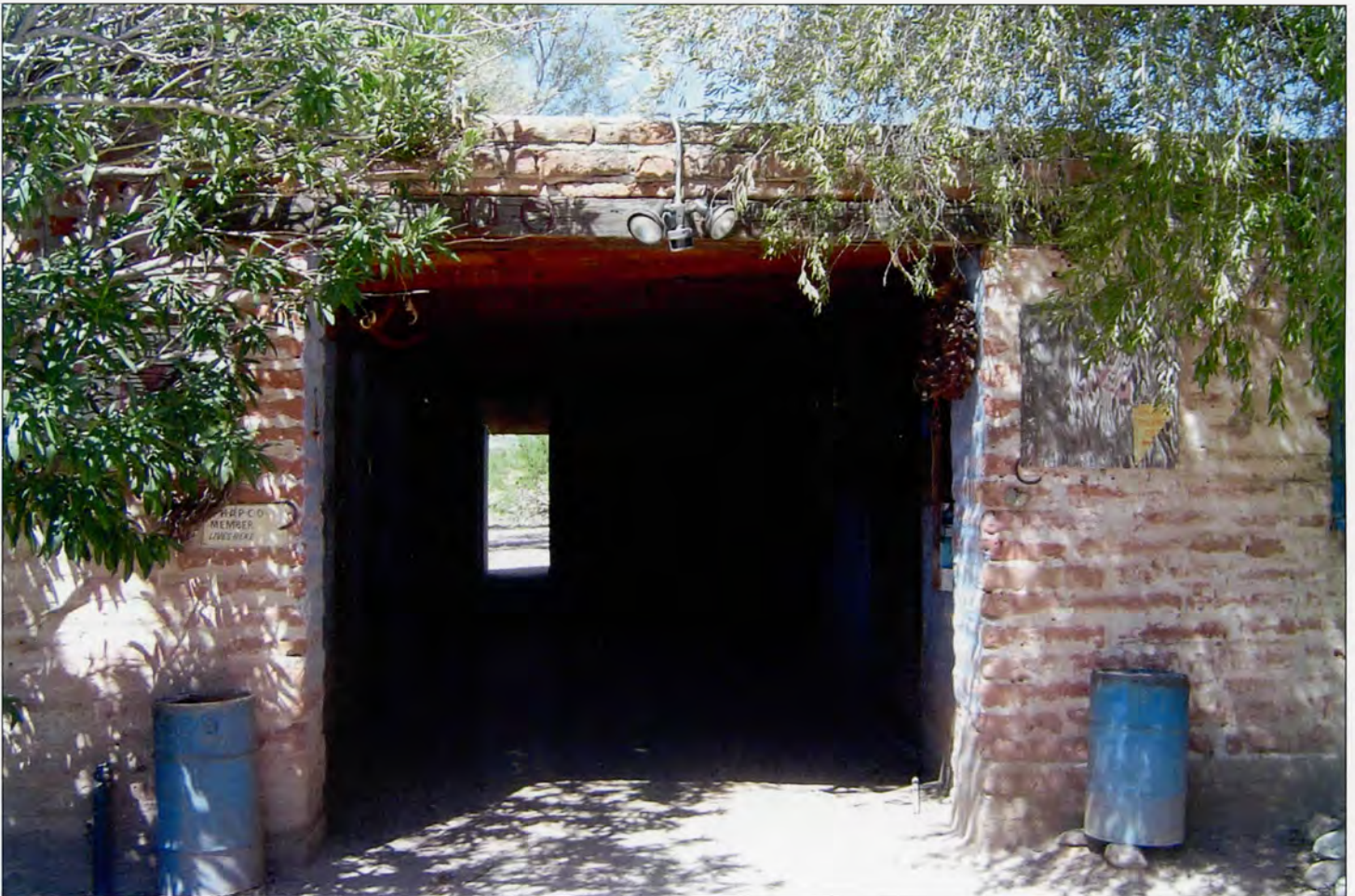
PHOTO #11: Stables facing west showing the east entrance, 4/2008
