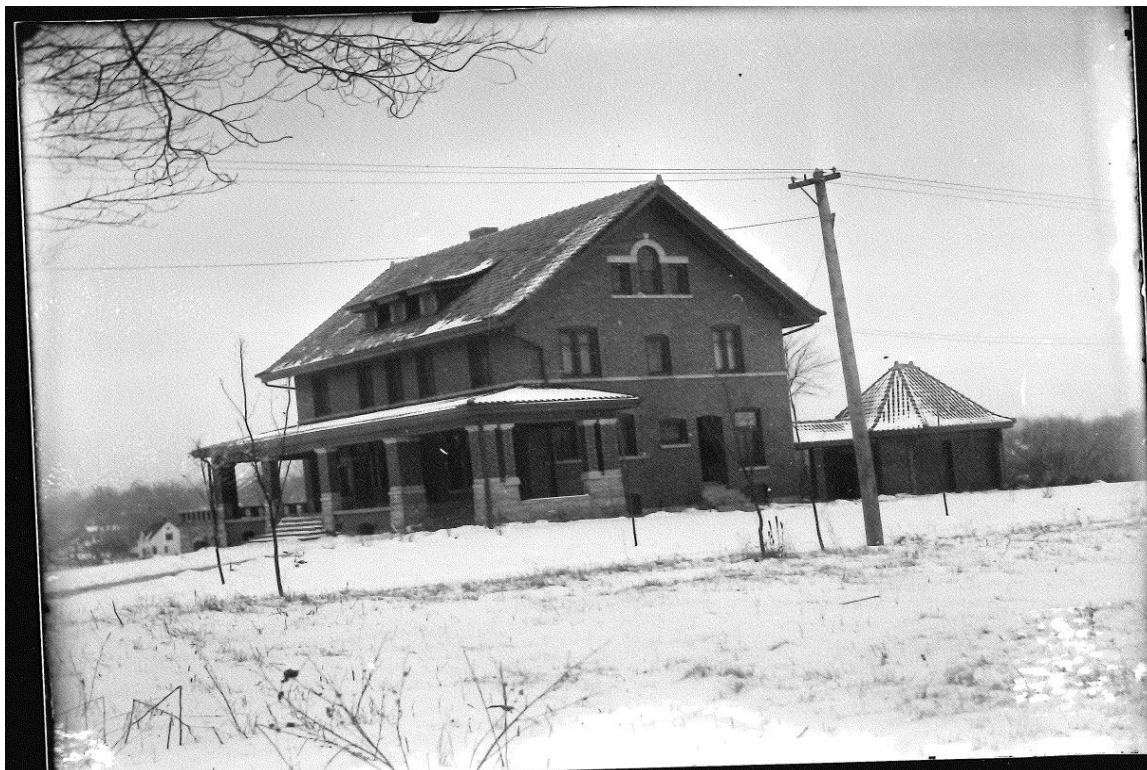
Figure 1 Home, carriage house, and grounds prior to wall's construction (1906)
