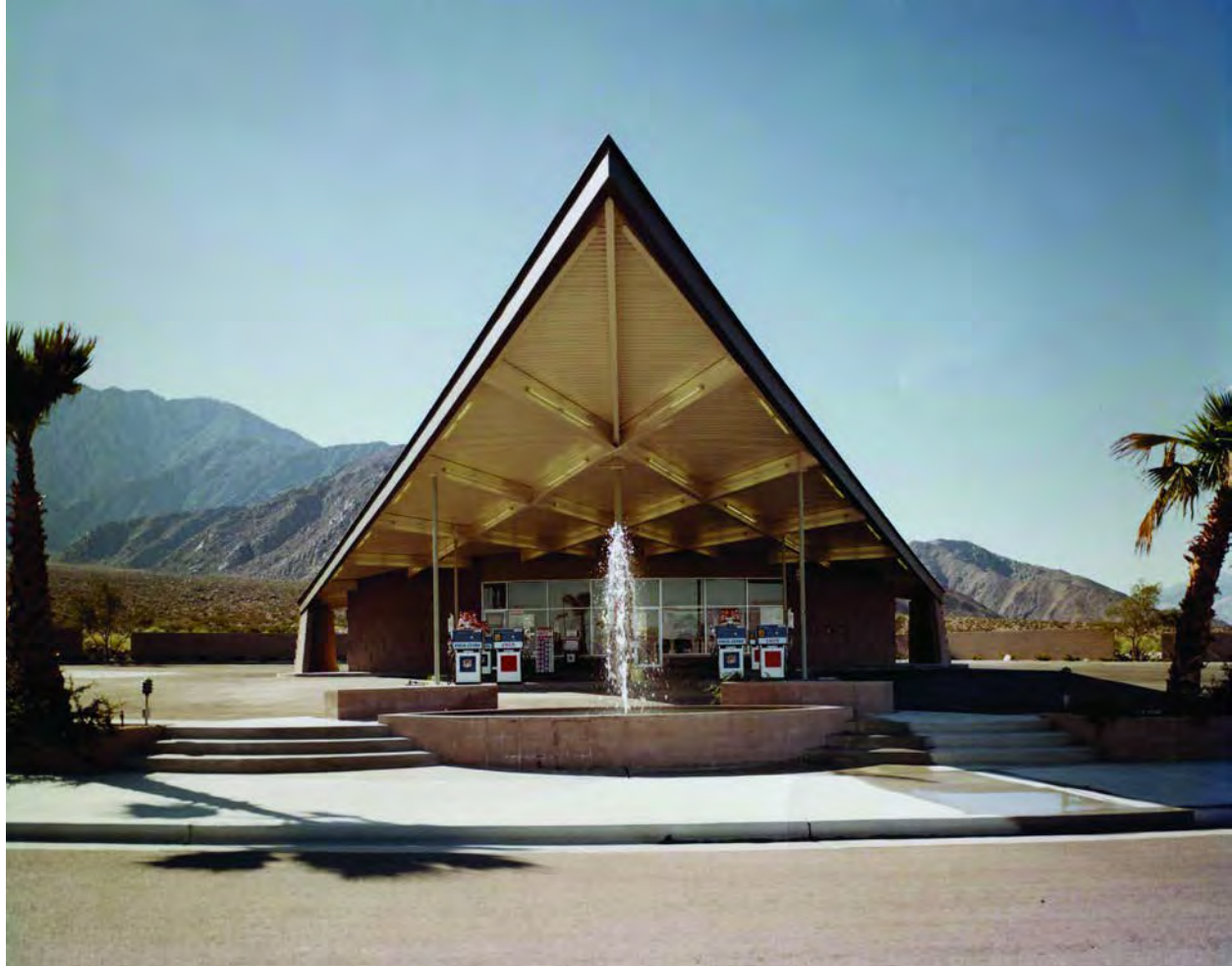
Figure 2. Southeast elevation, looking northwest, circa 1966. Photo courtesy Palm Springs Historical Society.
