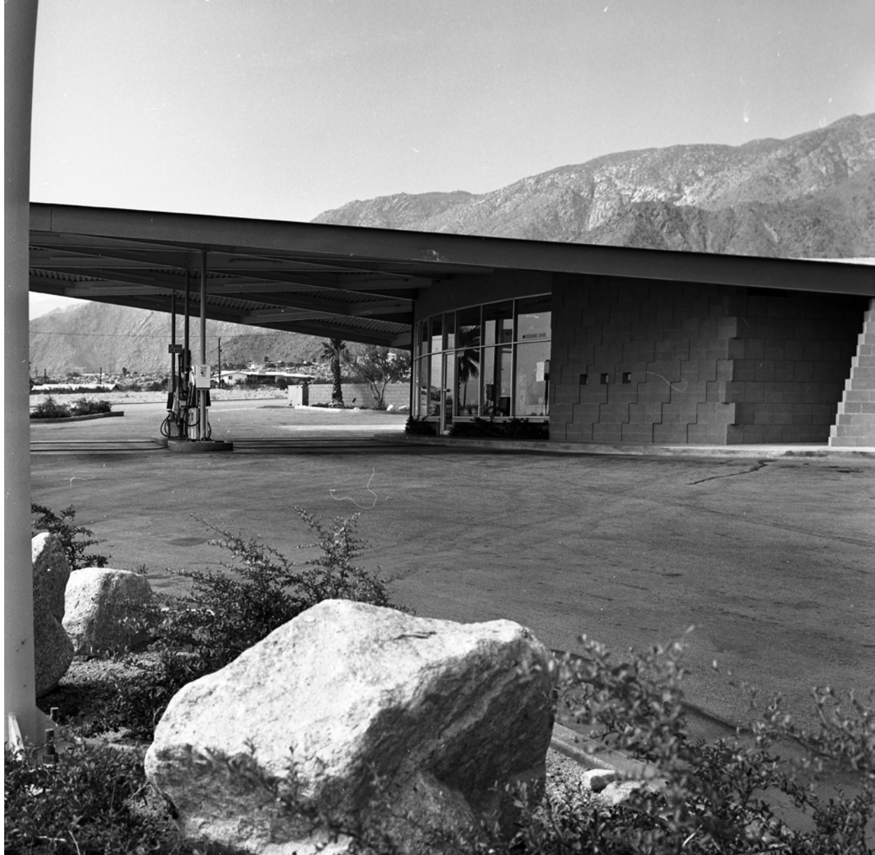
Figure 3. Northeast elevation, looking south, circa 1966. Photo courtesy Palm Springs Historical Society.
