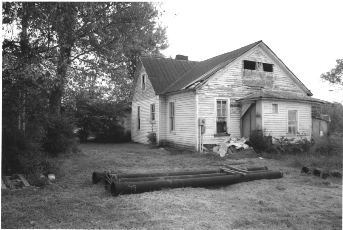
CHESNUTT, JAMES W. HOUSE McMINN COUNTY
