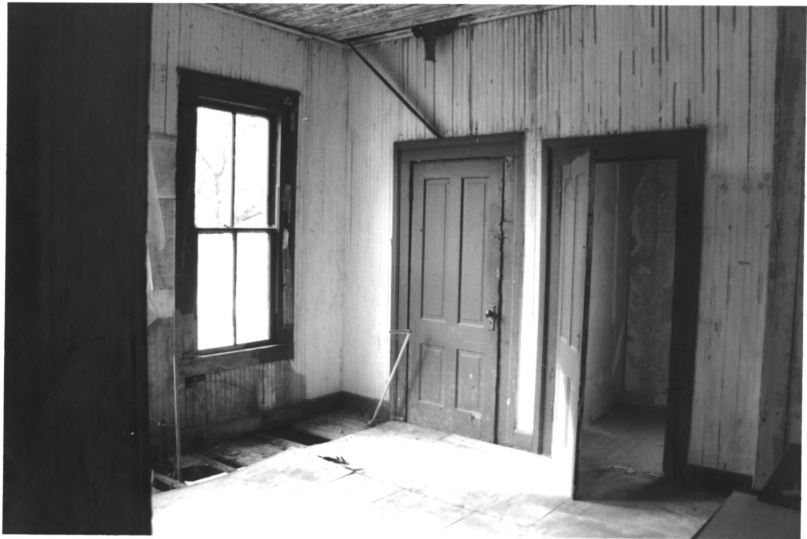
CHESNUTT, JAMES W. HOUSE McMINN COUNTY
