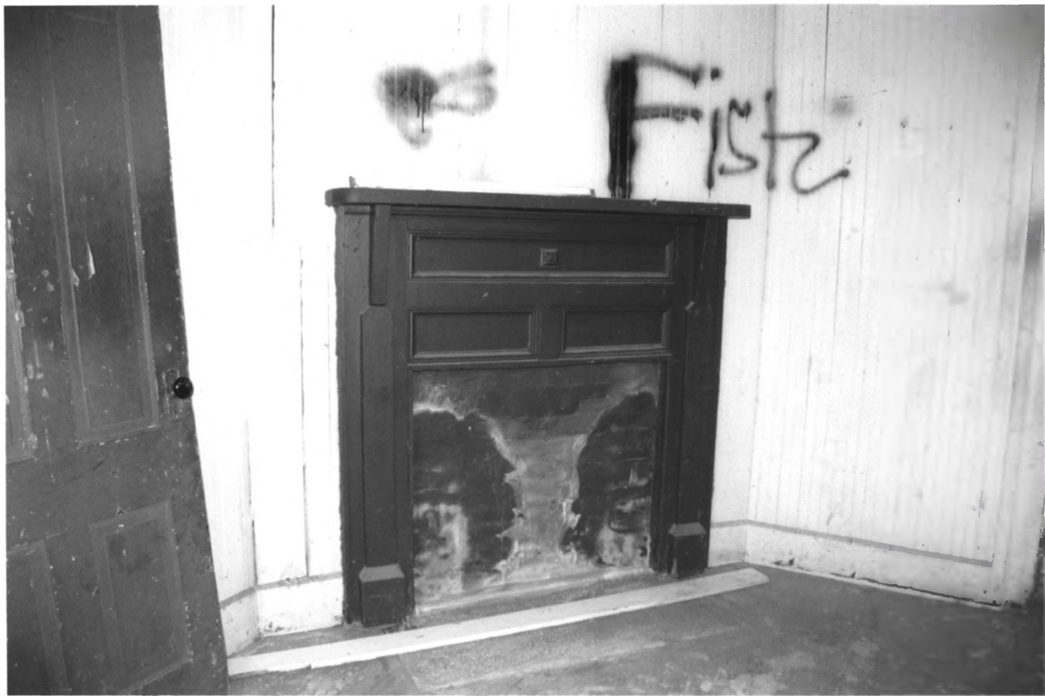
CHESNUTT, JAMES W. HOUSE McMINN COUNTY
