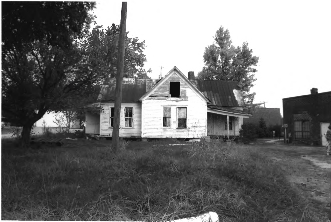
CHESNUTT, JAMES W. HOUSE McMINN COUNTY
