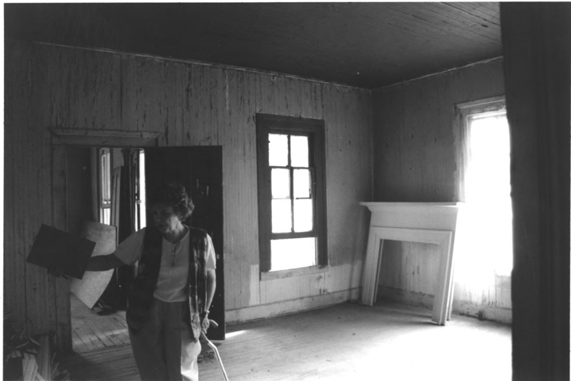
CHESNUTT, JAMES W. HOUSE McMINN COUNTY
