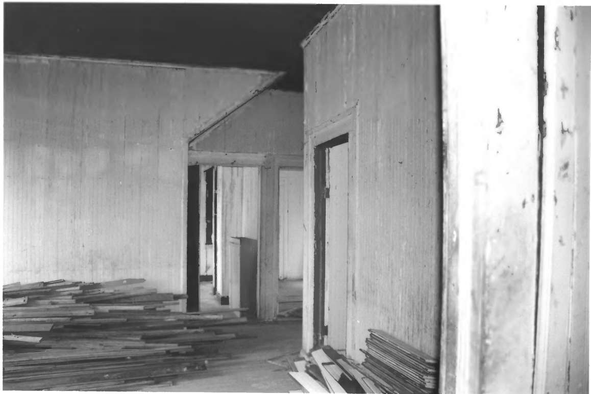
CHESNUTT, JAMES W. HOUSE McMINN COUNTY
