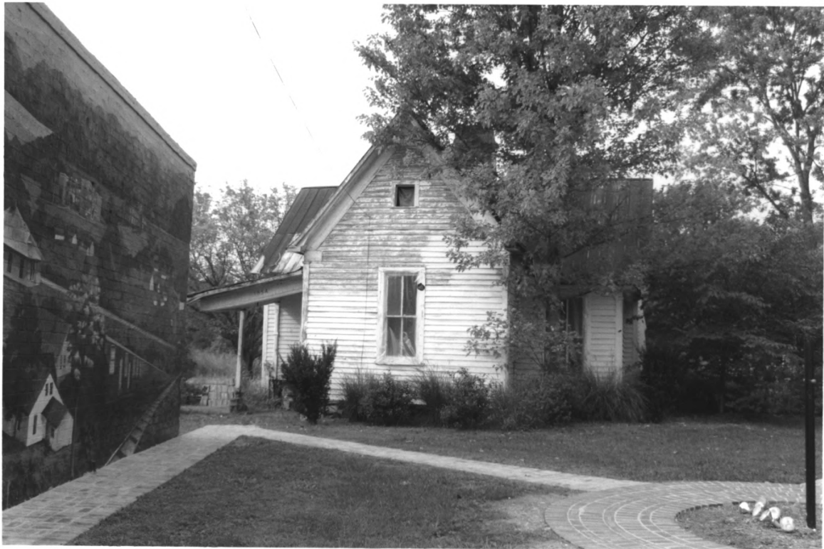
CHESNUTT, JAMES W. HOUSE McMINN COUNTY
