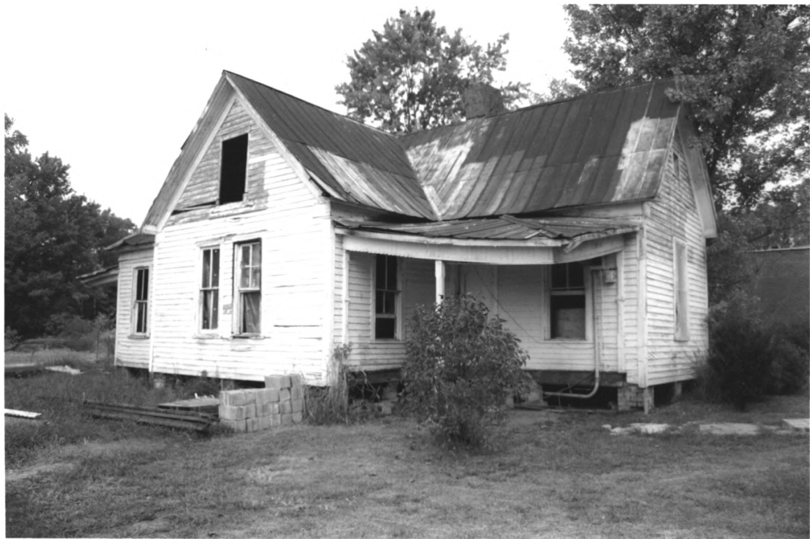
CHESNUTT, JAMES W. HOUSE McMINN COUNTY
