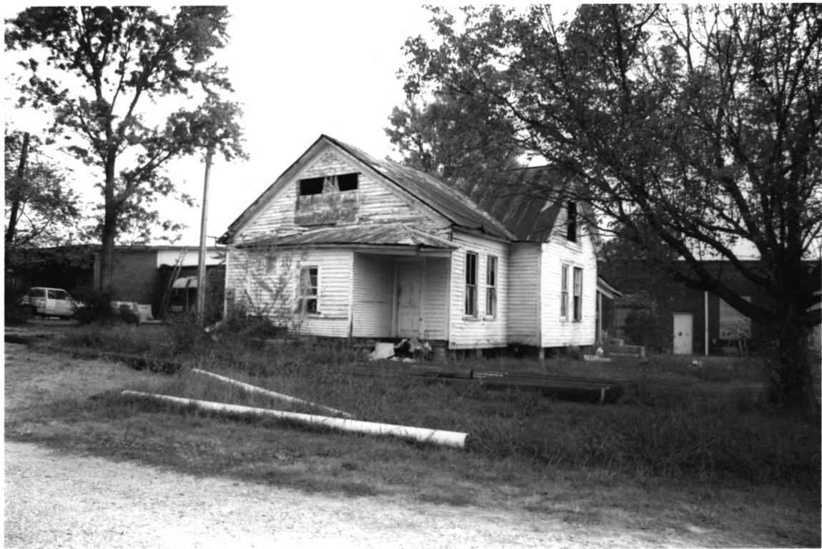
CHESNUTT, JAMES W. HOUSE McMINN COUNTY
