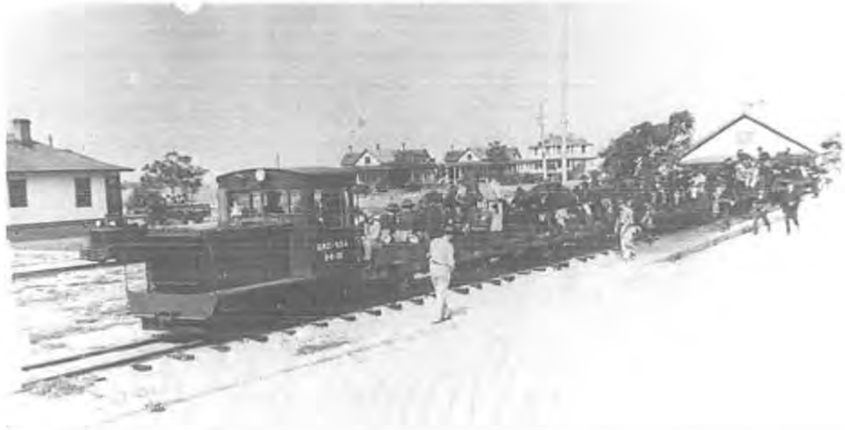
Figure 10. Fort Pickens rail line, 1941. The buildings visible in this photo include (from left to right): Building 1 (Non-commissioned Officers' Duplex, originally Firemen's Quarters), 1910; Buildings 2 and 3 (Lieutenant's Quarters), 1900; Building 4 (Captain's Quarters), 1912; and the Non-commissioned Officers' Quarters (as shown 1945 D-1 map). Photographer unknown; photograph courtesy of National Park Service, Gulf Islands National Seashore, catalogue no. 866.
