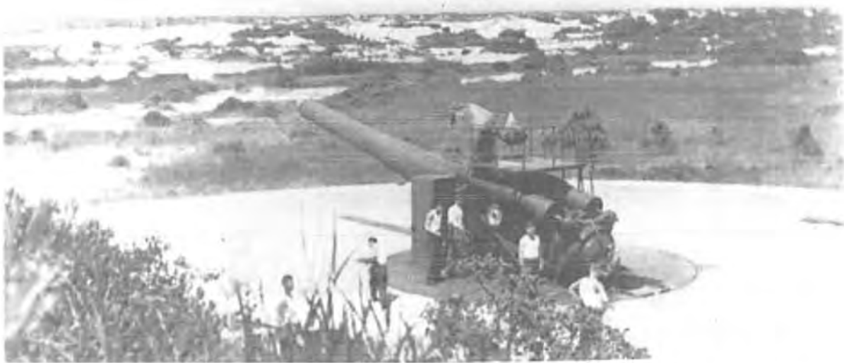
Figure 12. Battery Langdon circa 1939–1941, prior to encasement of the batteries in 1942–1943. Photographer unknown; photograph courtesy of National Park Service, Gulf Islands National Seashore, catalogue no. 17154.
