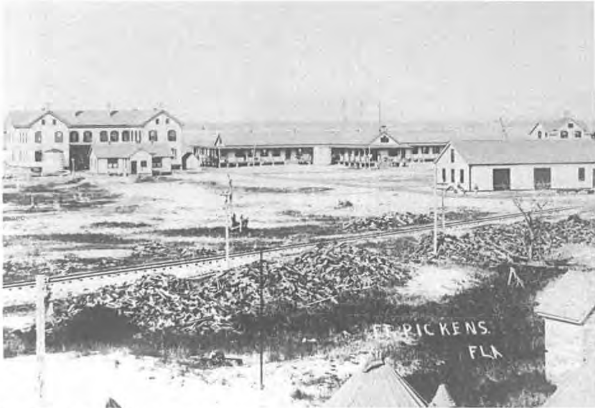
Figure 3. Fort Pickens looking toward the quarters and the mess hall (later the administration building), circa 1911. Two of the duplex quarters for officers are visible in the right background; the mess hall is in the center background; and a two-story barracks for enlisted men, with nearby latrine, is in the left background. The ordnance storeroom is visible in the right middle ground and the rail line is visible in the foreground. The enlisted barracks, latrine, and ordnance storeroom were later salvaged; the other buildings remain. Photograph courtesy of National Park Service, Gulf Islands National Seashore, from the Stillion Collection, catalogue no. 54906.
