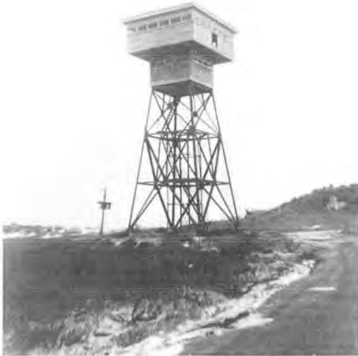
Figure 16. The Battery 234 Coincidence Range Finder/Battery Commander's Station Tower as completed, photograph dated August 26, 1946. Photographer unknown; photograph courtesy of National Park Service, Gulf Islands National Seashore, catalogue no. 946.
