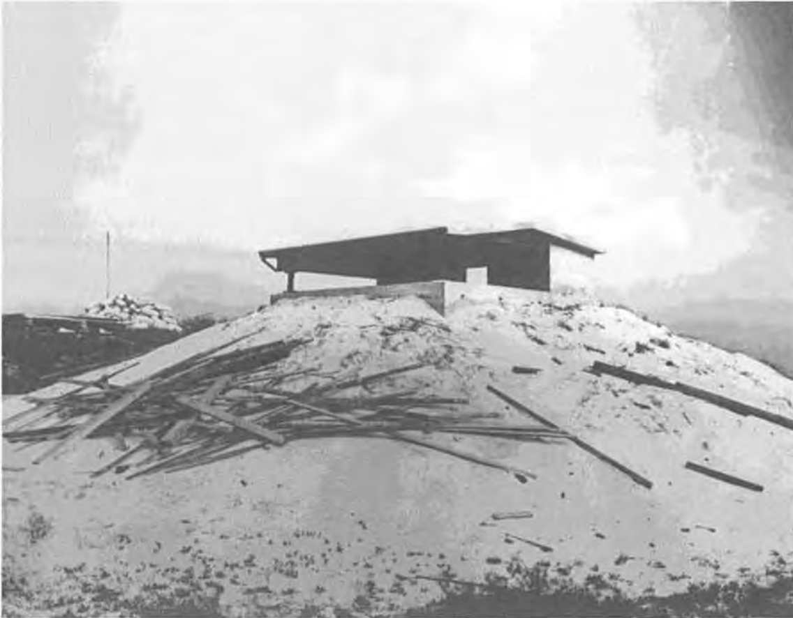
Figure 7. Battery Trueman, Battery Commander's Station, circa 1922. Photographer unknown; National Archives Record Group 77, File 600.92; photograph courtesy of National Park Service, Gulf Islands National Seashore, catalogue no. 634.
