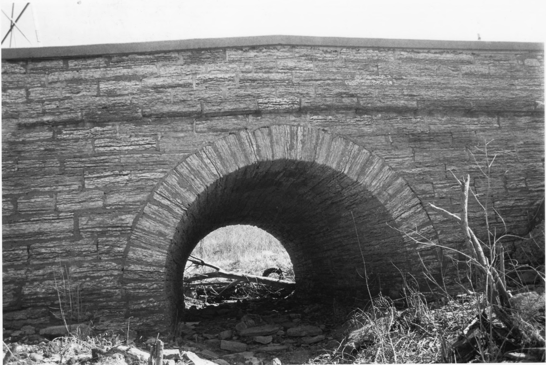
MENDOTA ROAD BRIDGE (NO. 90401) RAMSEY CO., MN. PHOTO I.D. 09739 #8
