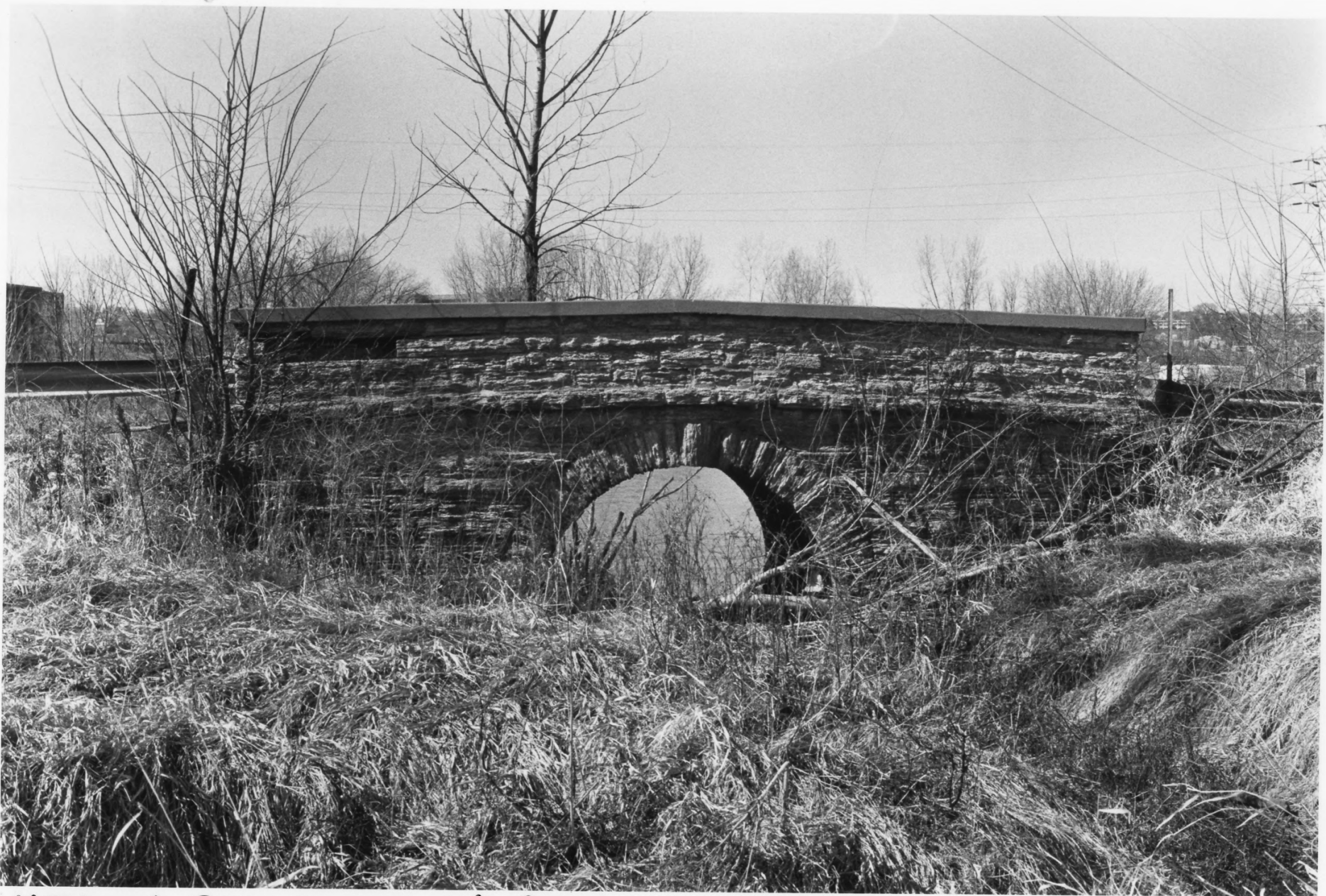
MENDOTA ROAD BRIDGE (NO. 90401) RAMSEY CO., MN PHOTO I.D. 09739#4
