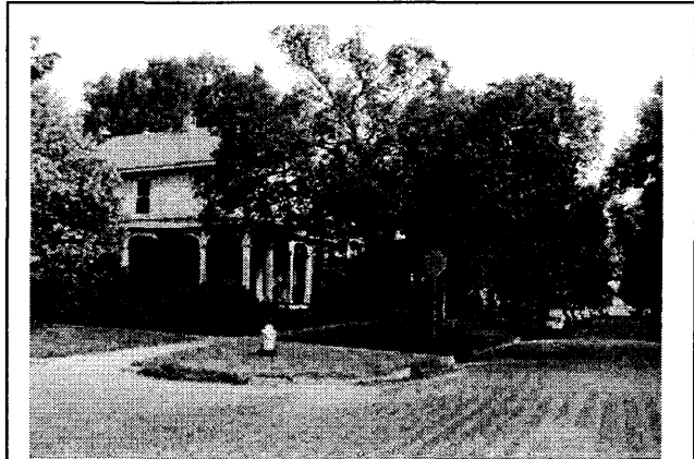
900 Block (west side) Rhode Island Street, Looking North from 10 th Street (Photo #30)
