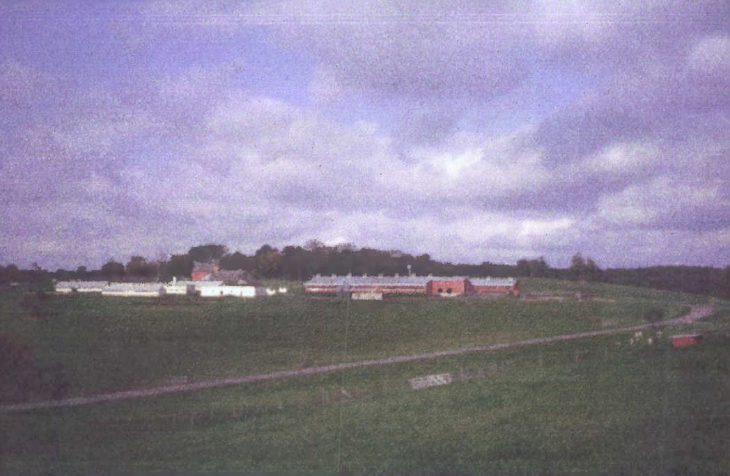
Photo 9. Distant view northwest from the top of Horse Barn Hill across Agricultural School fields and farm buildings to Farwell Barn. (scanned version only).
