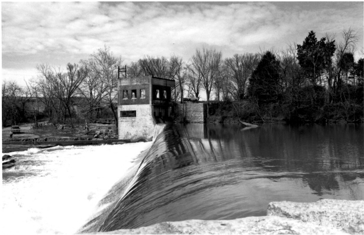
Walter Hill Hydroelectric Station Murfreesboro, Rutherford Co., TN
