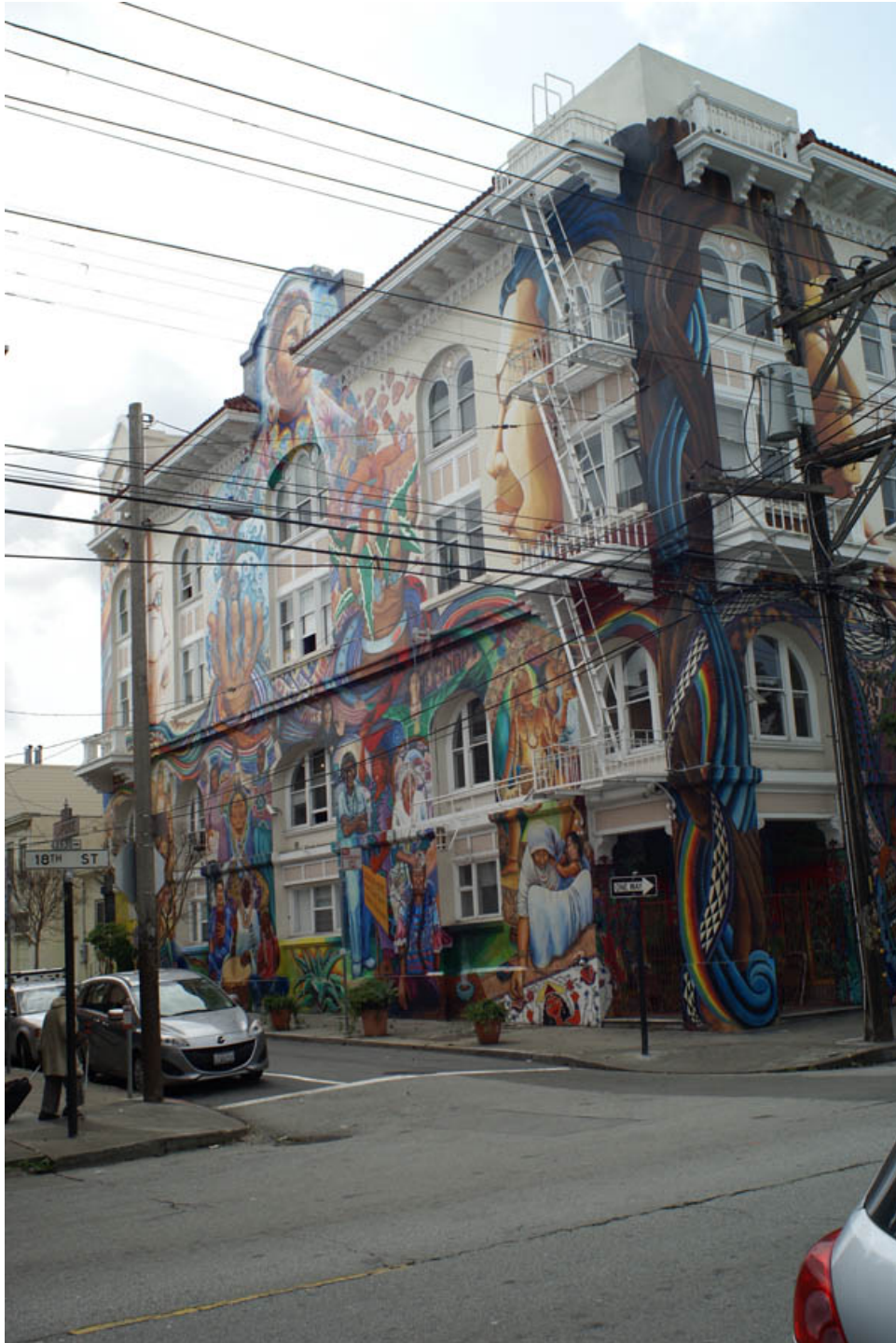
Photo 2. East façade, looking southwest.
