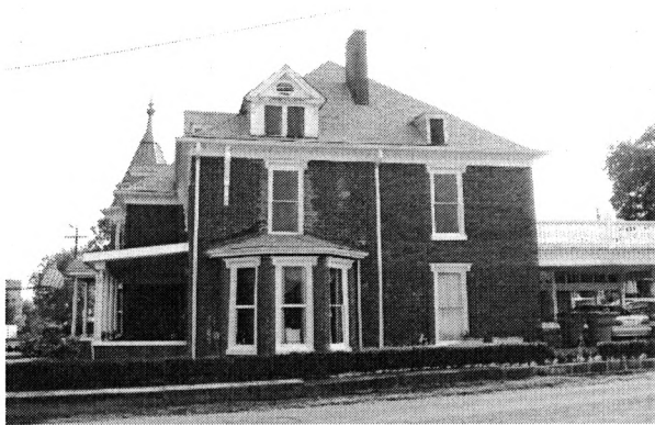
North Elevation, View to the South
