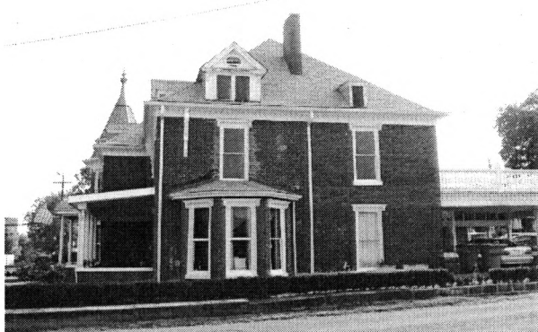
North Elevation, View to the South
