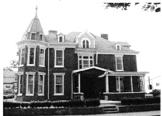
East Façade, View to the West
