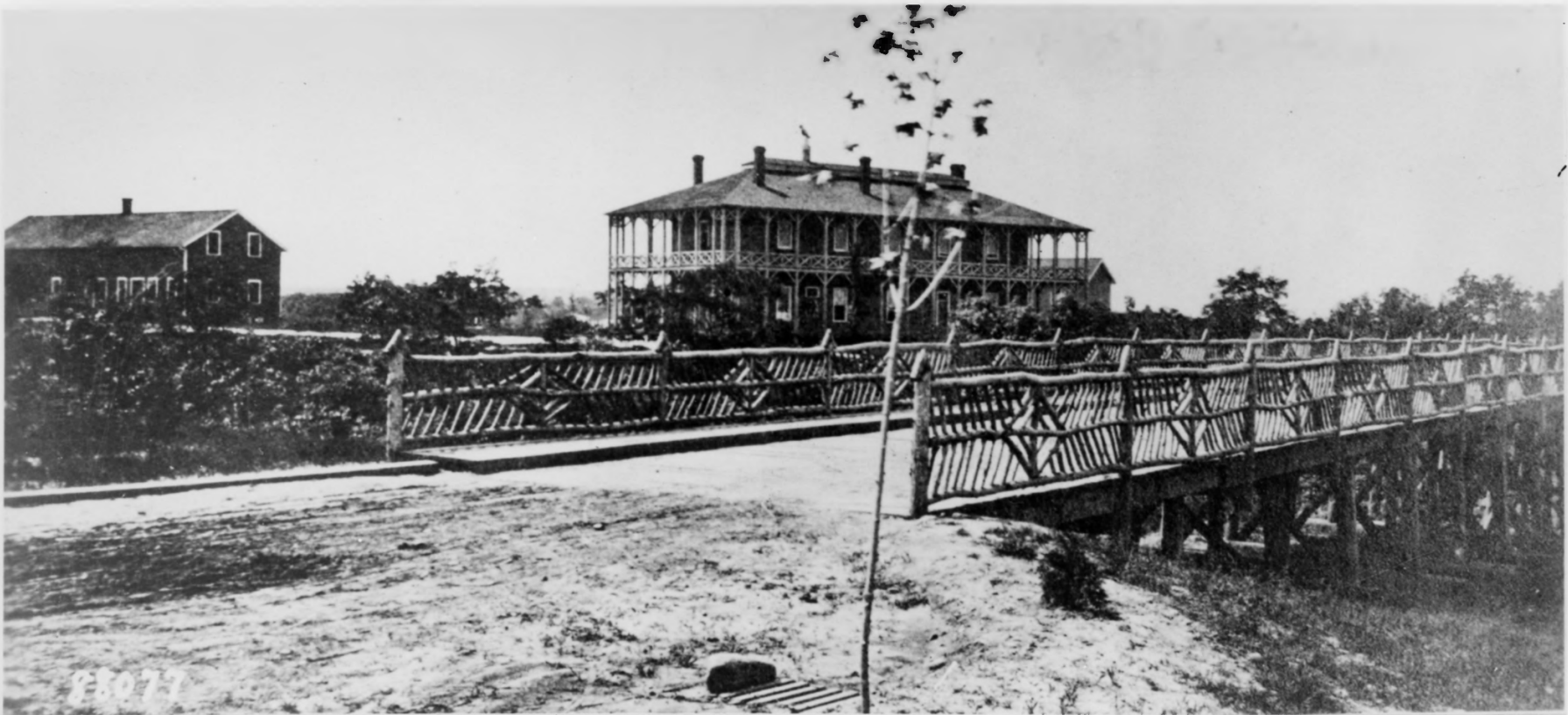
Fort Myer, Virginia--Old Post Hospital in 1876.
