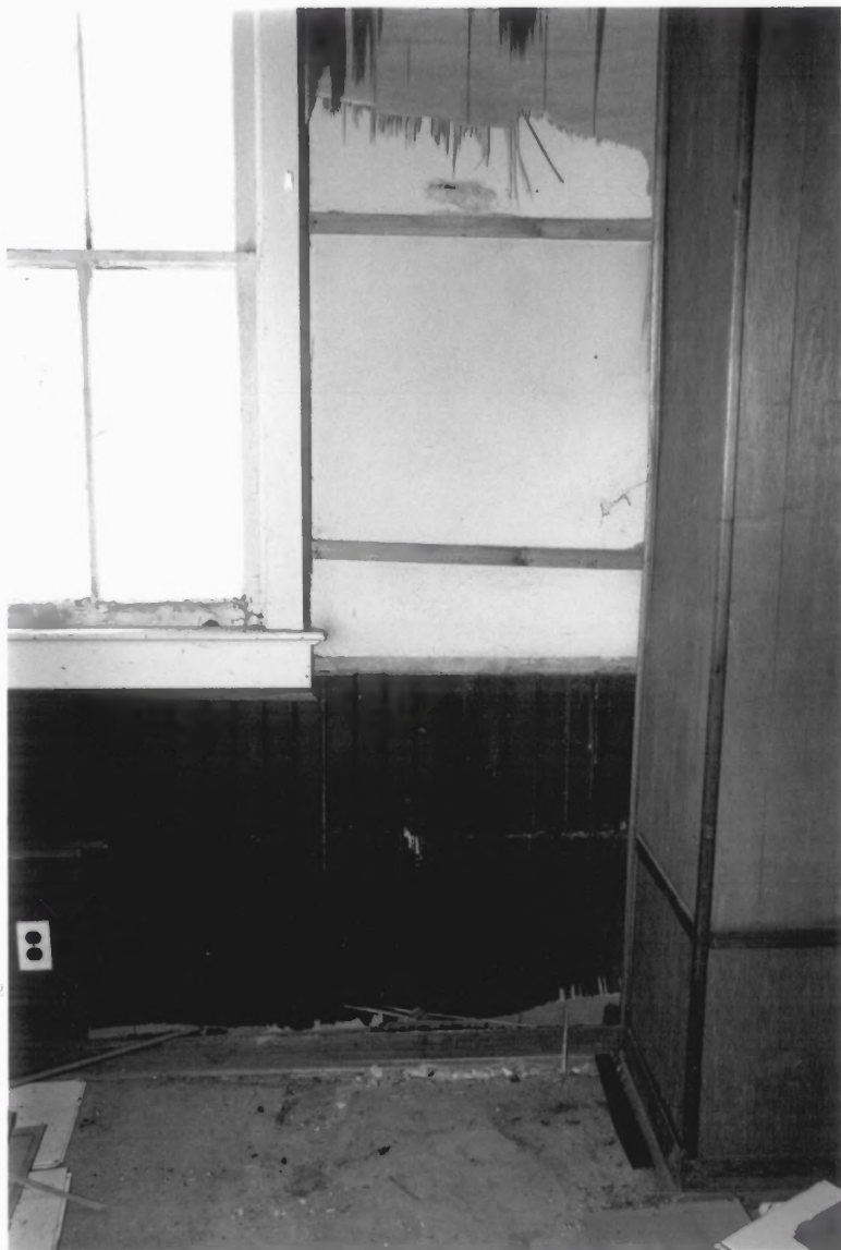
CARPENTER STREET SCHOOL GLOUCESTER CO, NJ PHOTO 8 OF 9
