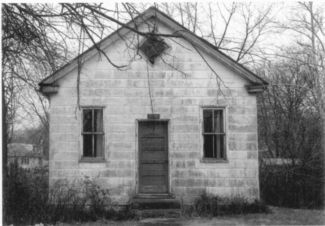
CARPENTER STREET SCHOOL GLOUCESTER CO, MA PHOTO 2 OF 9
