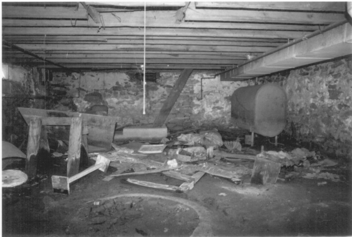
CARPENTER STREET SCHOOL GLOUCESTER CO, NJ PHOTO 9 OF 9
