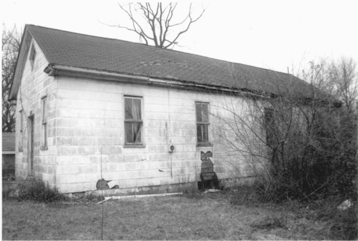
CARPENTER STREET SCHOOL GLOUCESTER CO., NJ PHOTO 3 OF 9
