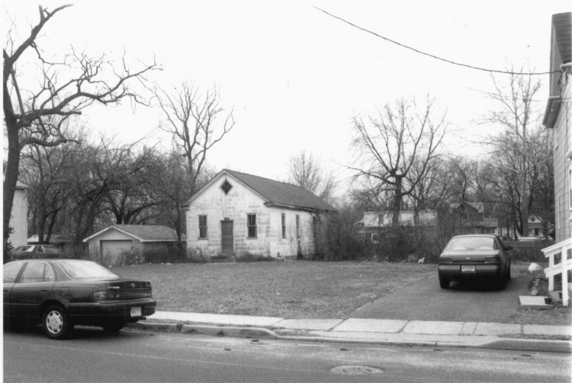
CARPENTER STREET SCHOOL GLOUCESTER CO., NJ PHOTO 1 OF 9
