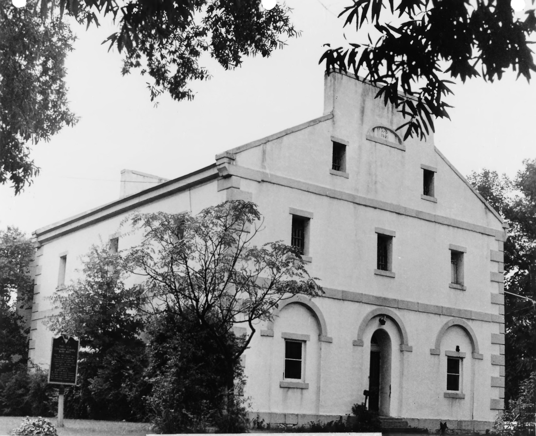
Lancaster County Jail, South Carolina
