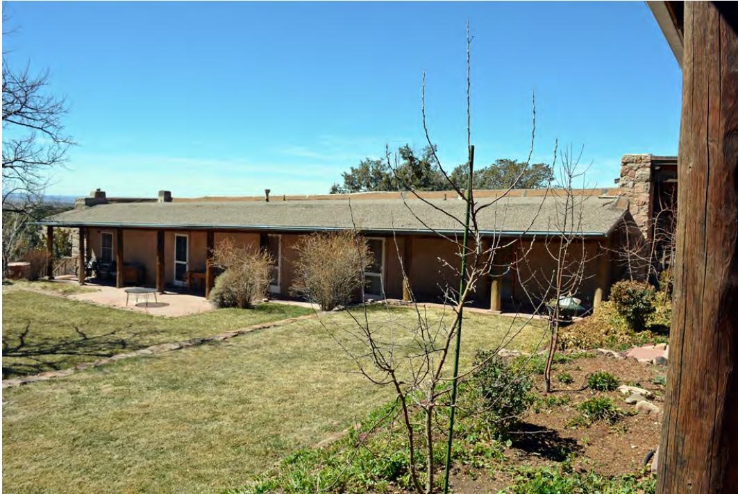
Photo 3 of 30: Preexisting Building (West Wing), east elevation, facing southwest.
