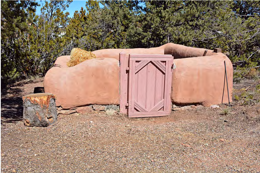
Photo 29 of 30: Trash incinerator, facing northwest.
