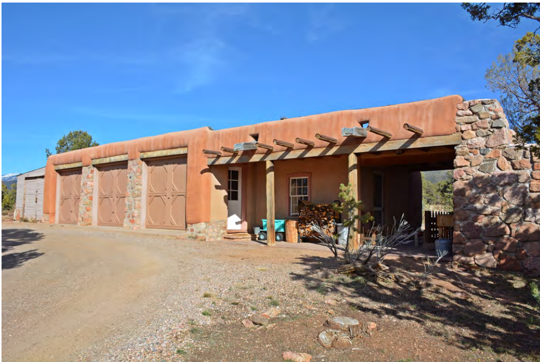
Photo 22 of 30: Service Area (Northeast Wing), garage, west elevation, facing northeast.
