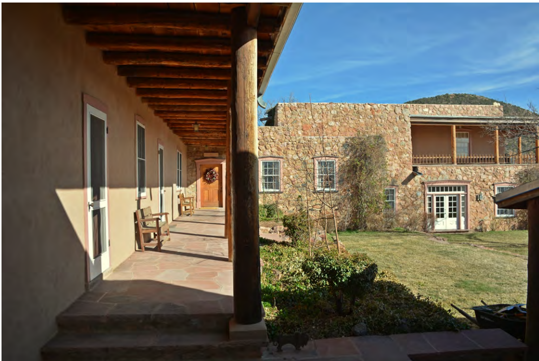
Photo 10 of 30: Entry Portal (North Wing), facing east. Sections 9-end page 49
