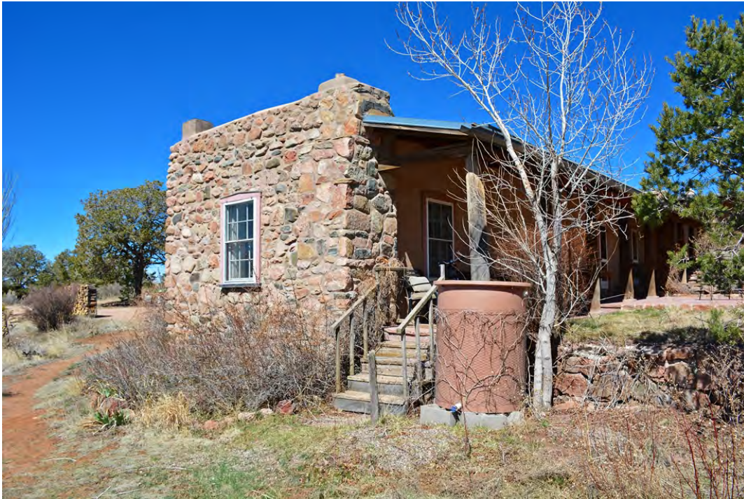
Photo 5 of 30: Preexisting Building (West Wing), south and east elevations, facing northwest.
