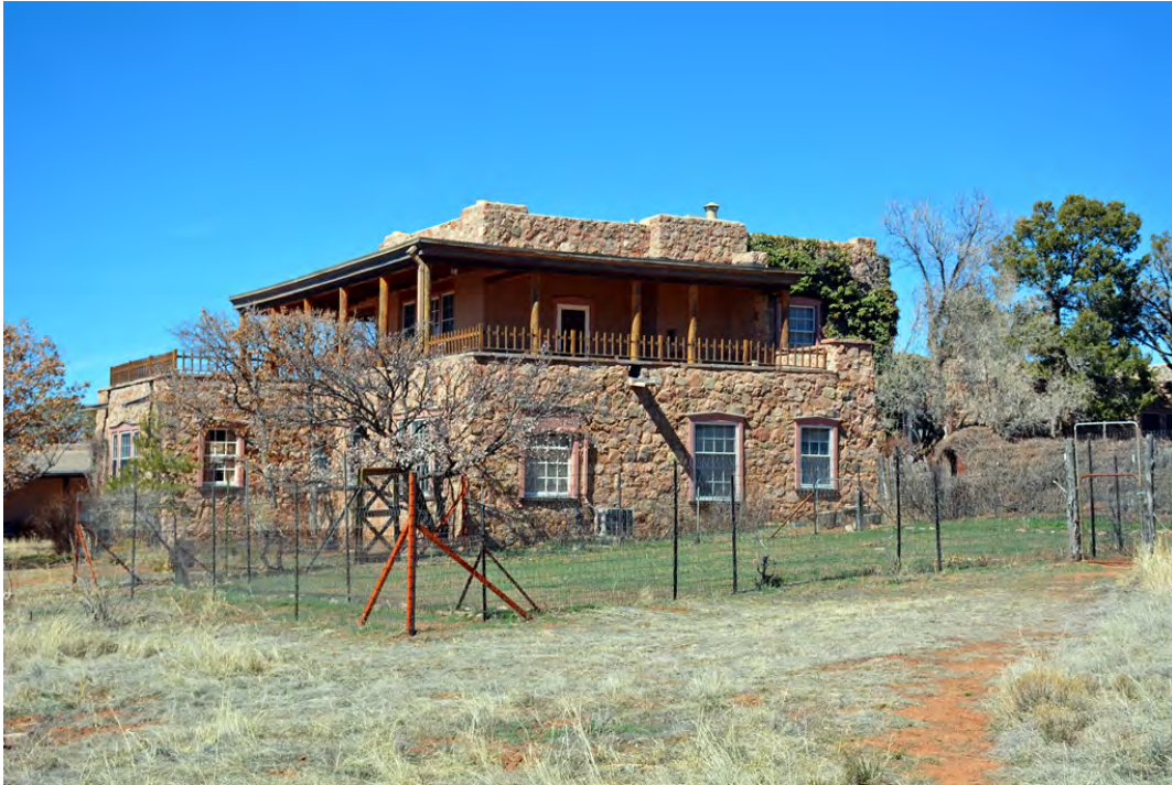
Photo 13 of 30: Main House (East Wing), south and east elevations, facing northwest.
