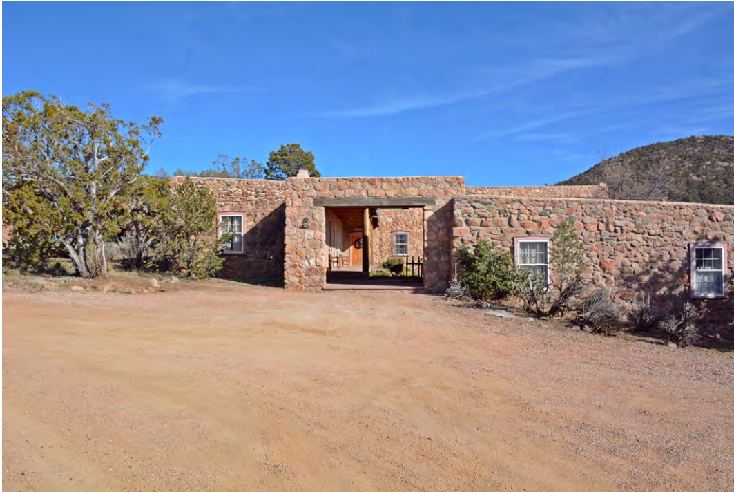
Photo 7 of 30: Partial west elevation, with zaguan at center, facing southeast.
