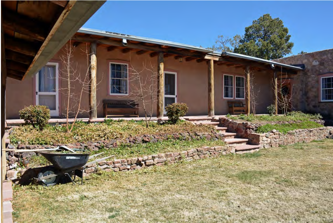
Photo 11 of 30: Entry Portal (North Wing), facing northeast.
