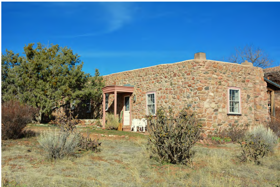
Photo 2 of 30: Preexisting Building (West Wing), west and south elevations, facing northeast.
