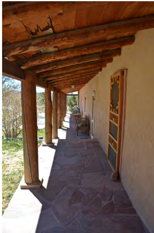
Photo 4 of 30: Preexisting Building (West Wing), east elevation portal, facing southwest.
