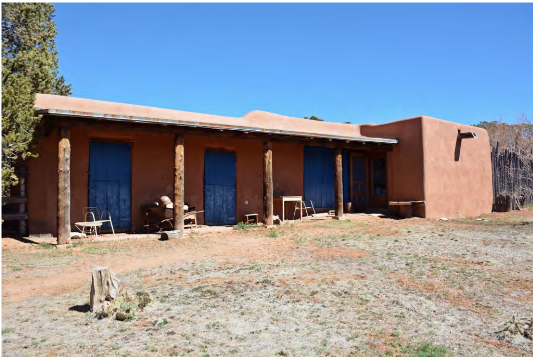
Photo 26 of 30: Stable/Barn/Tack Room, south elevation, facing northeast.
