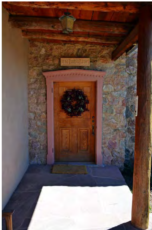
Photo 16 of 30: Main House (East Wing), entry door, facing southeast.
