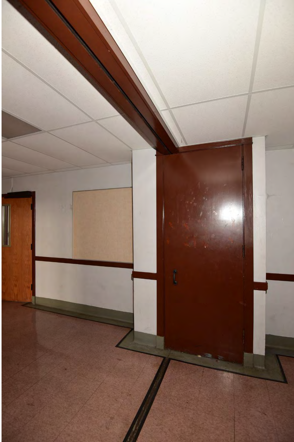
Figure 14. Seam between building campaigns. Source: Brad Finch, 2017.
