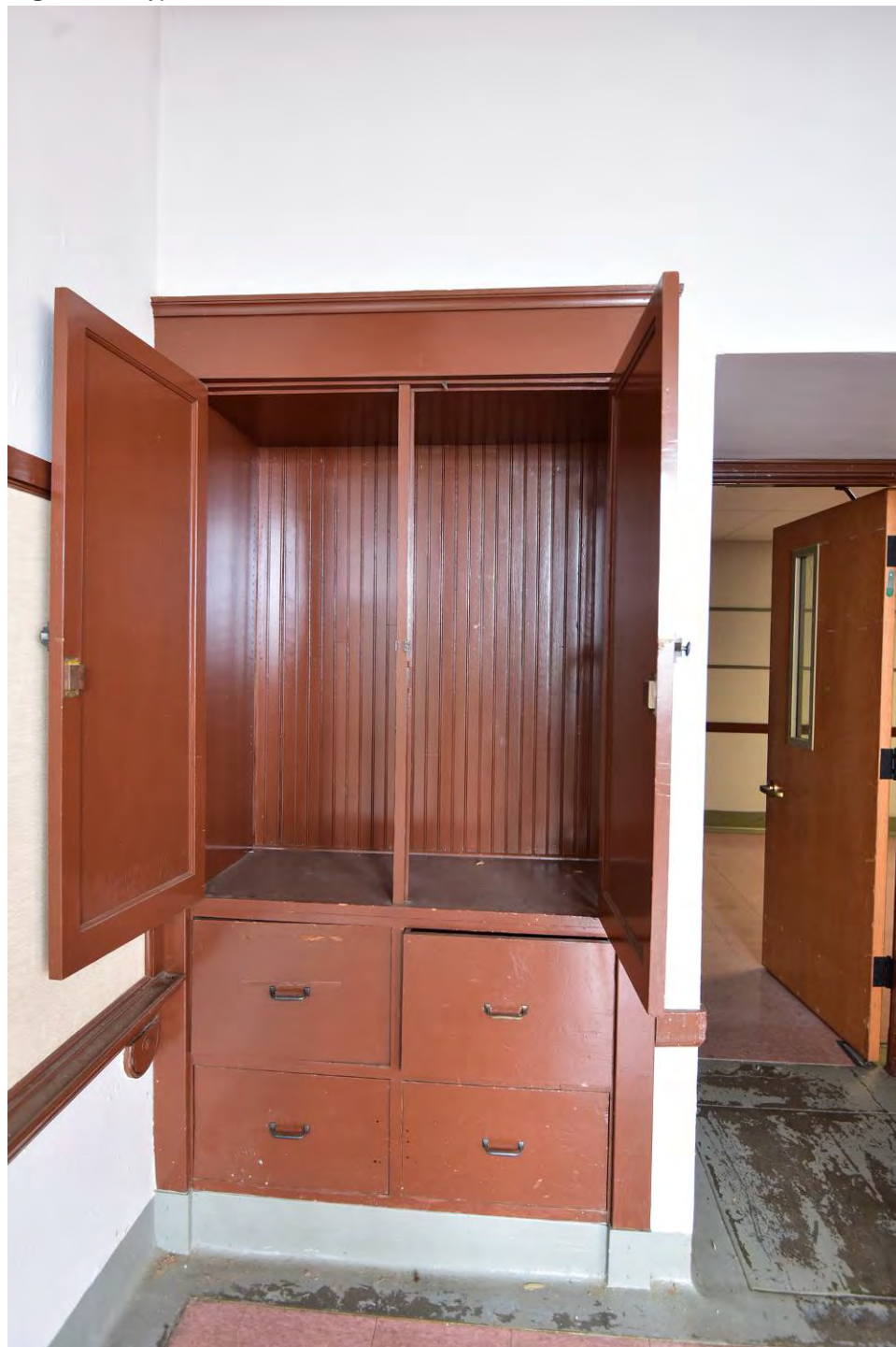
Figure 16. Typical built-in cabinets. Source: Brad Finch, 2017.
