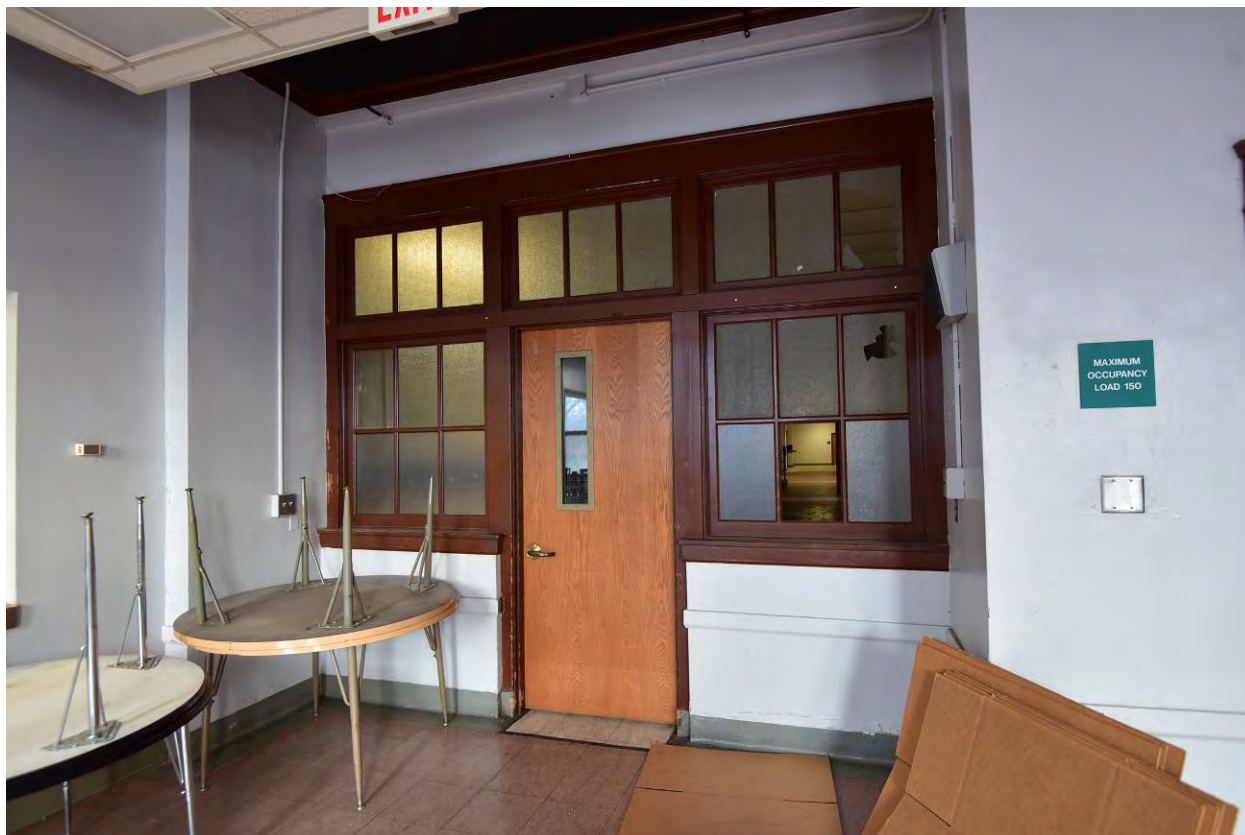
Figure 17. Historic windows that provided borrowed light for the Fresh Air Classroom. Source: Brad Finch, 2017.
