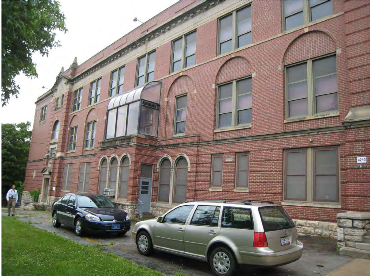
Figure 25. Meservey School, primary elevation. Source: Rosin Preservation Staff, 2011.
