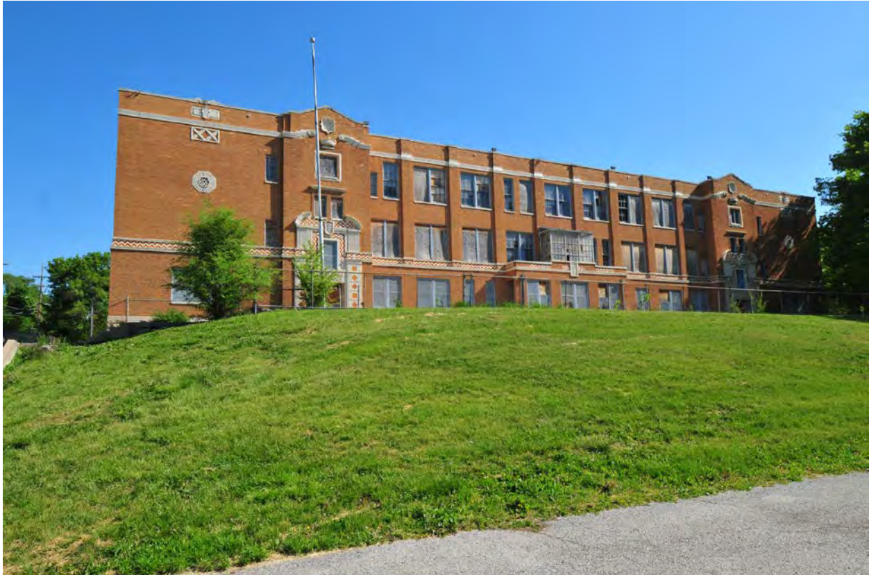
Figure 24. Seven Oaks School, primary elevation. Source: Brad Finch, 2012.
