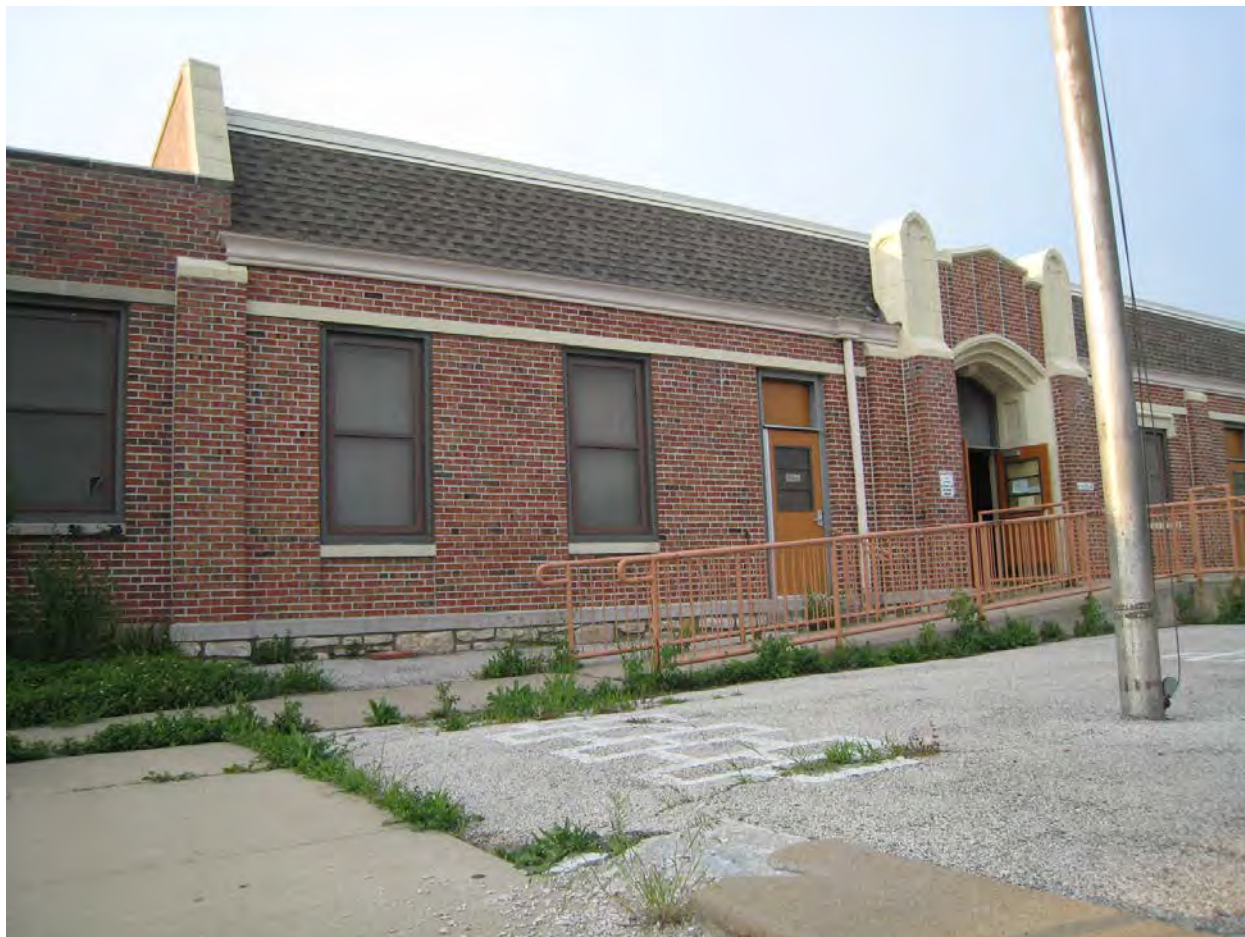
Figure 29. Askew School, south elevation. Source: Rosin Preservation Staff, 2011.
