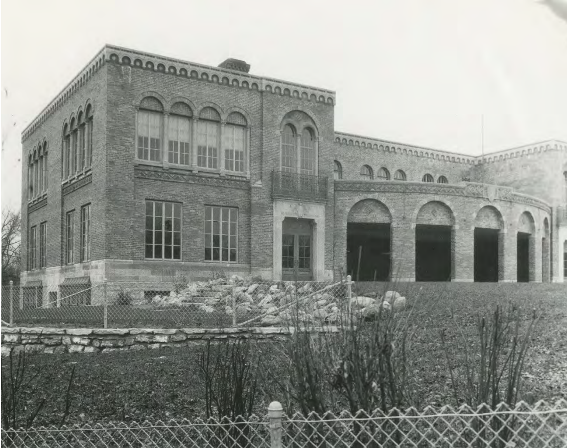
South and West Elevations 1928 Building Courtesy Columbus Metropolitan Library Historic Photograph Collection
