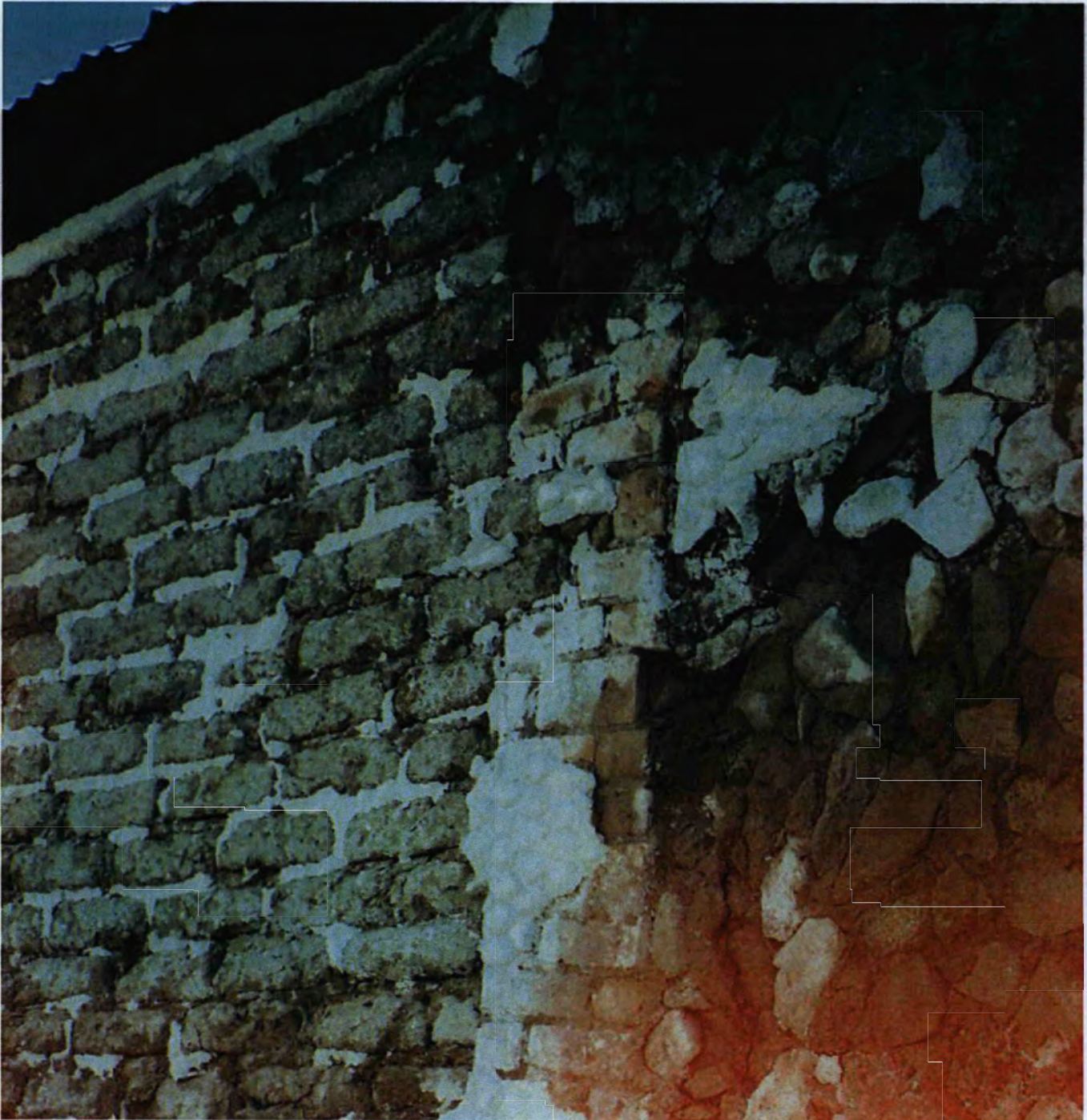
Figure 7. View of the joint exposed along the exterior west wall of the schoolhouse during the 1994 rehabilitation work (courtesy Mary Kasulaitis, Arivaca).
