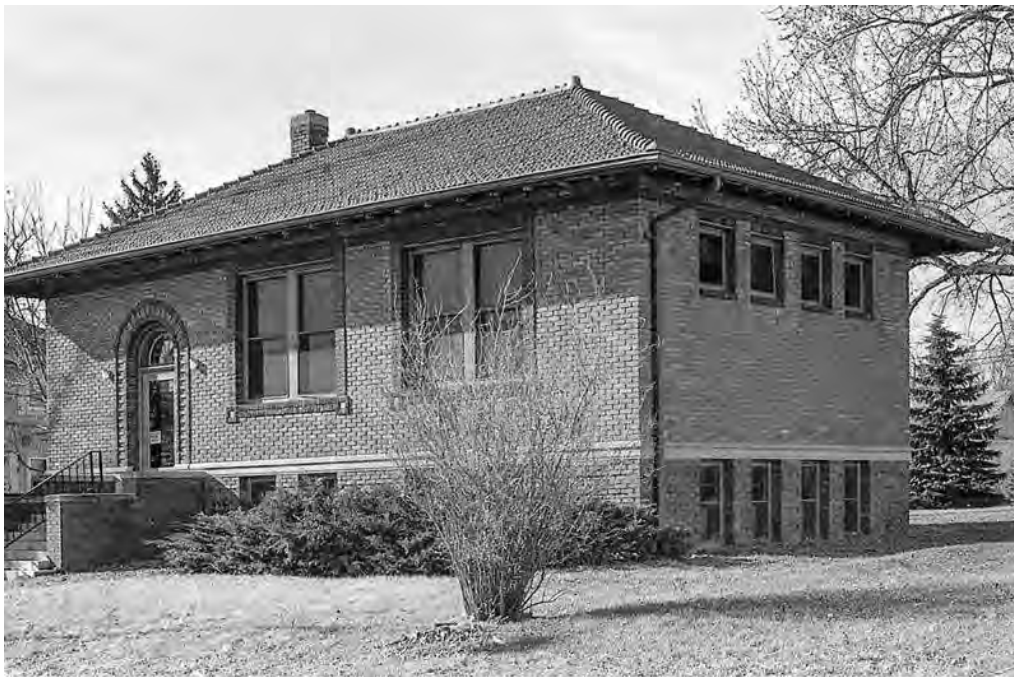
Figure 2: Hartington Carnegie Library pre-1998 addition, 1987. 3
