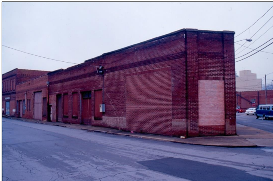
Figure 9: Building at the corner of King and Montgomery Streets in 2003. View is to the east.
