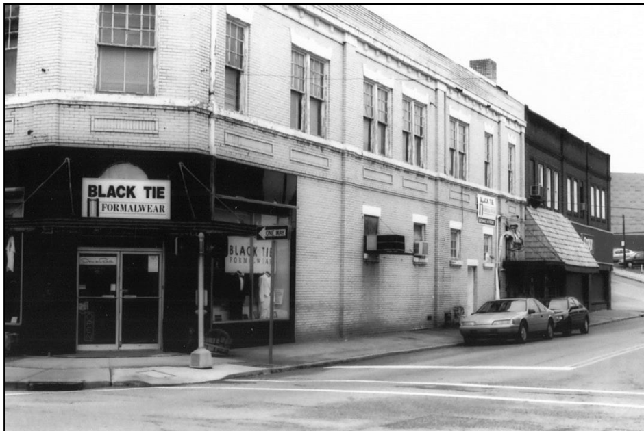
Figure 3: Streetscape of North Boone Street in 2003. View to the north-northwest.
