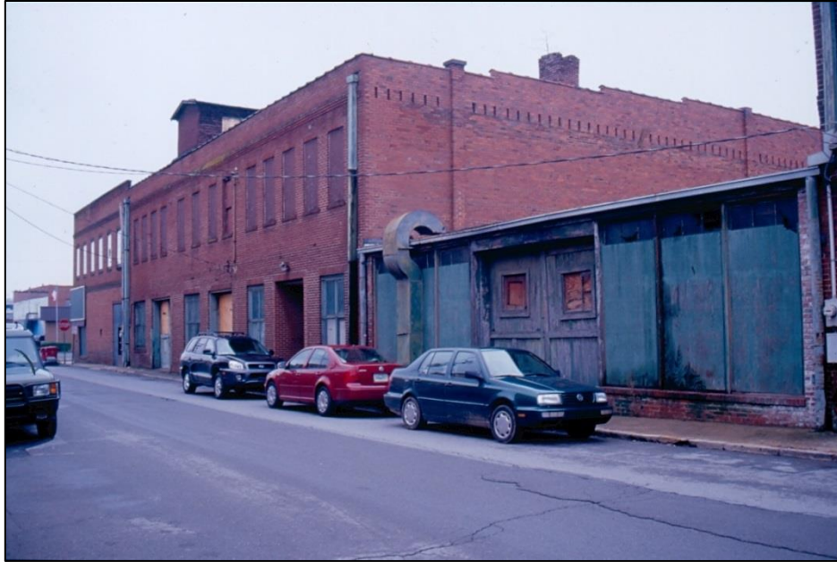
Figure 11: Rear elevations on King Street for the 204 and 210 West Market and the north elevation of 107 North Boone Street in 2003. View is to the east.
