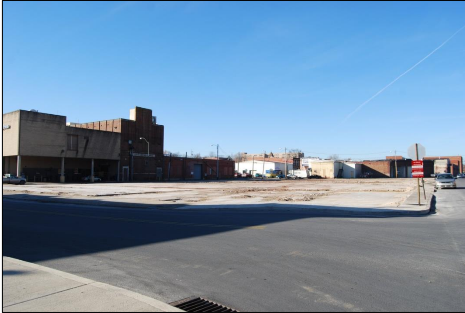
Figure 24: View to the west of the demolished block. Photo dated 12/06/2013.
