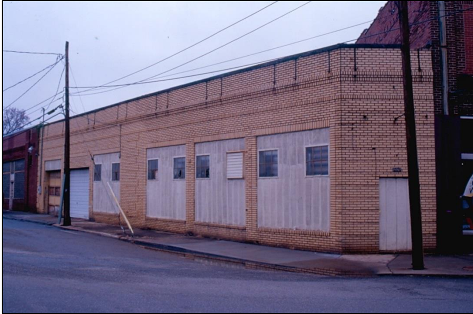
Figure 8: 200 West Market Street in 2003. View is to the east.
