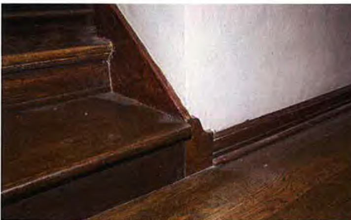
Photograph #14. Stairs between living room and dining room, camera facing west.
