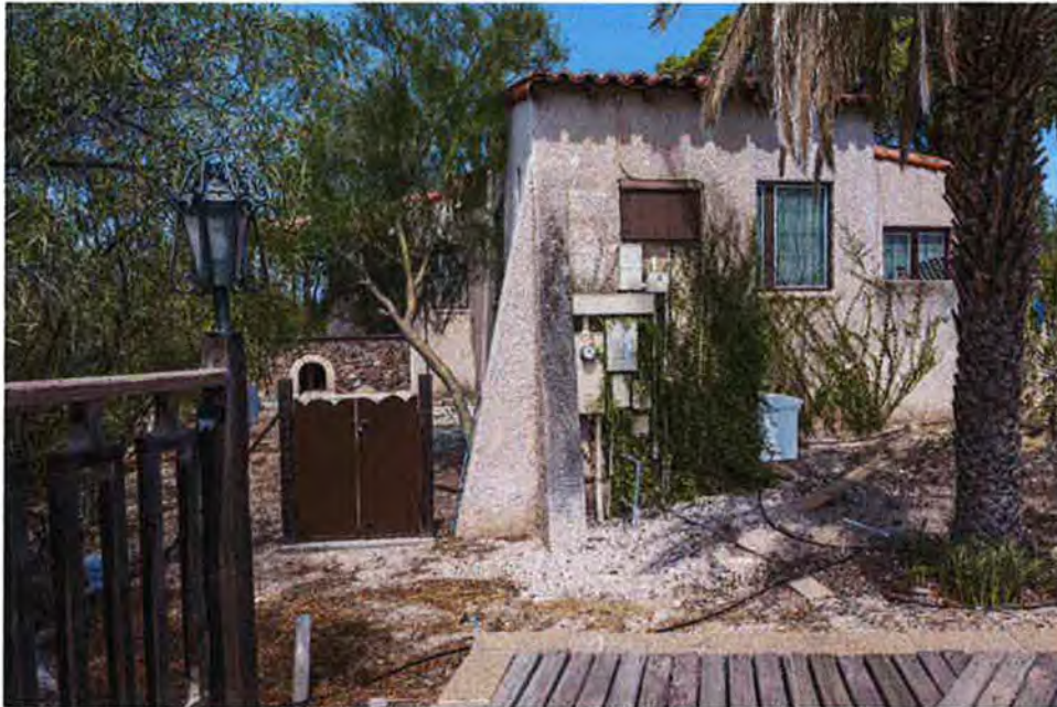
Photograph #7. Buttresses at southeast end of house, camera facing west.
