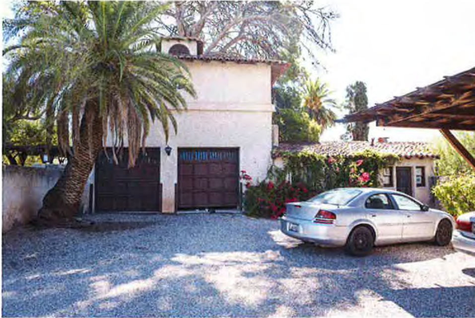
Photograph #9. West façade, camera facing southeast.
