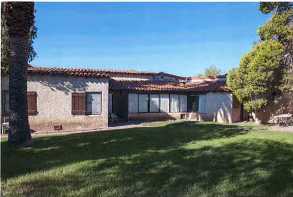
Photograph #10. North façade showing 1956 enclosed porch, camera facing southwest.
