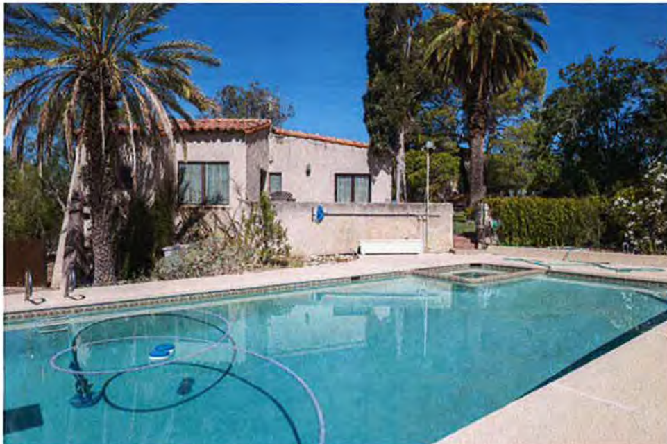
Photograph #8 East façade, camera facing west.
