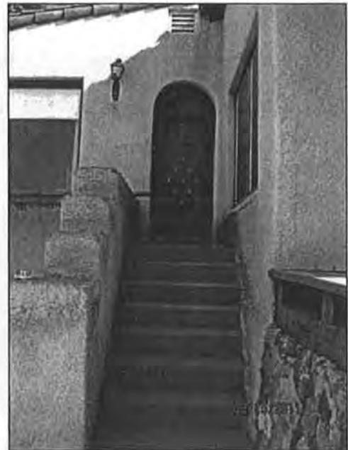
Photograph #6 Original entry and staircase, south façade, camera facing north.
