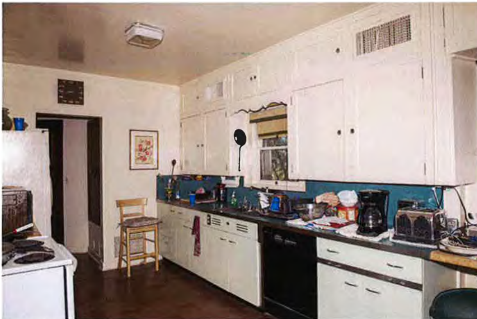
Photograph #18. St. Charles kitchen cabinets, camera facing southwest.
