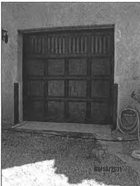
Photograph #7 Original wood-panel garage doors, camera facing northeast.
