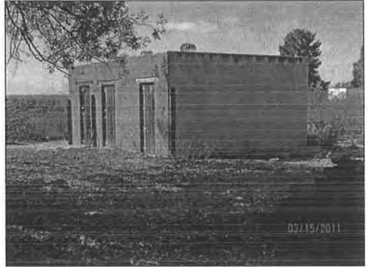
Photograph #10 Stable building, camera facing southwest.
