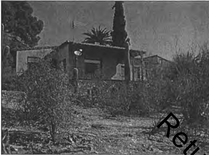
Photograph #5 Front (south) façade, camera facing northeast.
