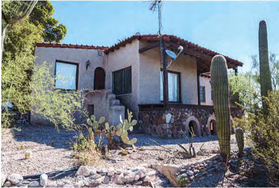
Photograph #5 South façade, camera facing northeast.
