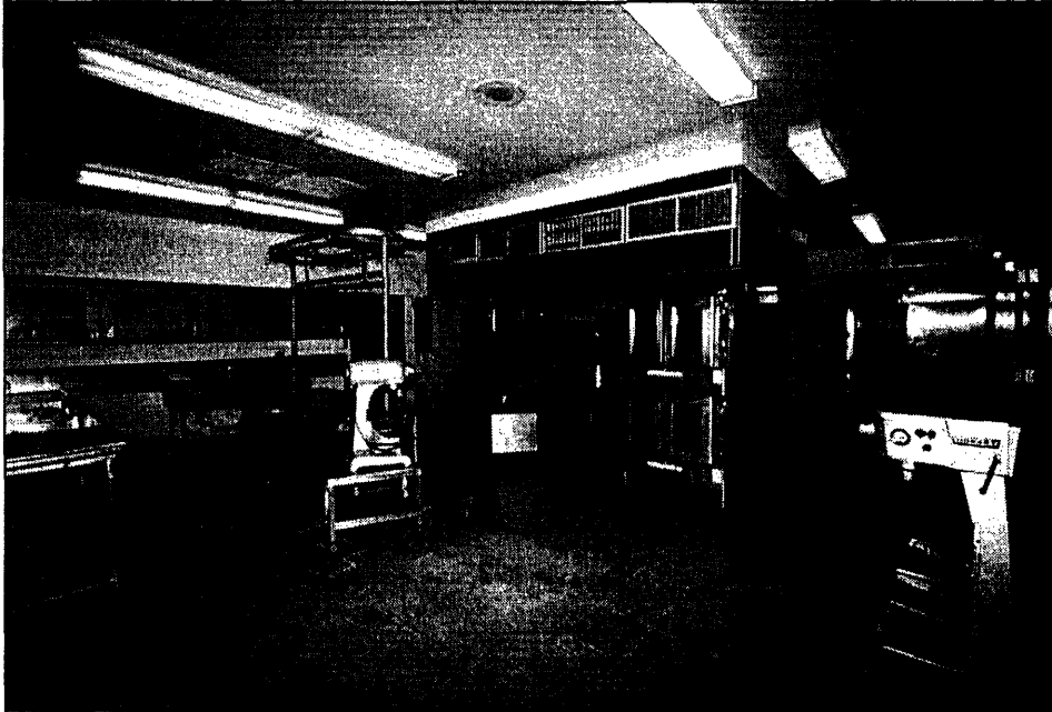
Kitchen, view looking south from northwest corner. The floor is tile. Beyond the southwest wall (left of picture) are large walk-in cold storage lockers.
