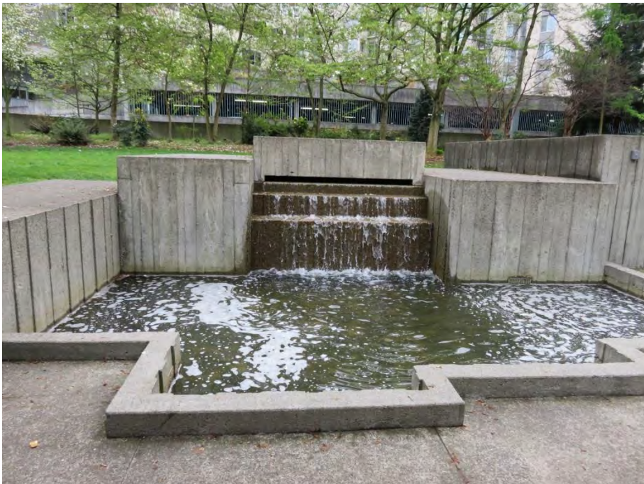
Photo 19 of 28. WA_King County_Freeway Park 0020. East Plaza Water Display, also known as the children's wading pool, view east.
