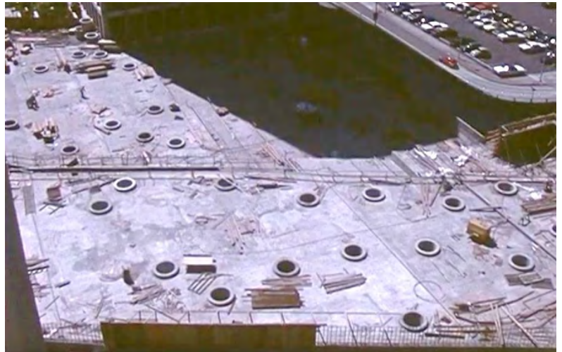
Freeway Park, view showing large tree wells. Image courtesy of Seattle Municipal Archives. Freeway Park and Garage (1st Phase)
