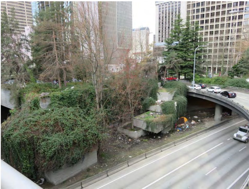
Photo 2 of 28. WA_King County_Freeway Park 0002. Freeway Park's Great Box Garden over I-5, view northwest.
