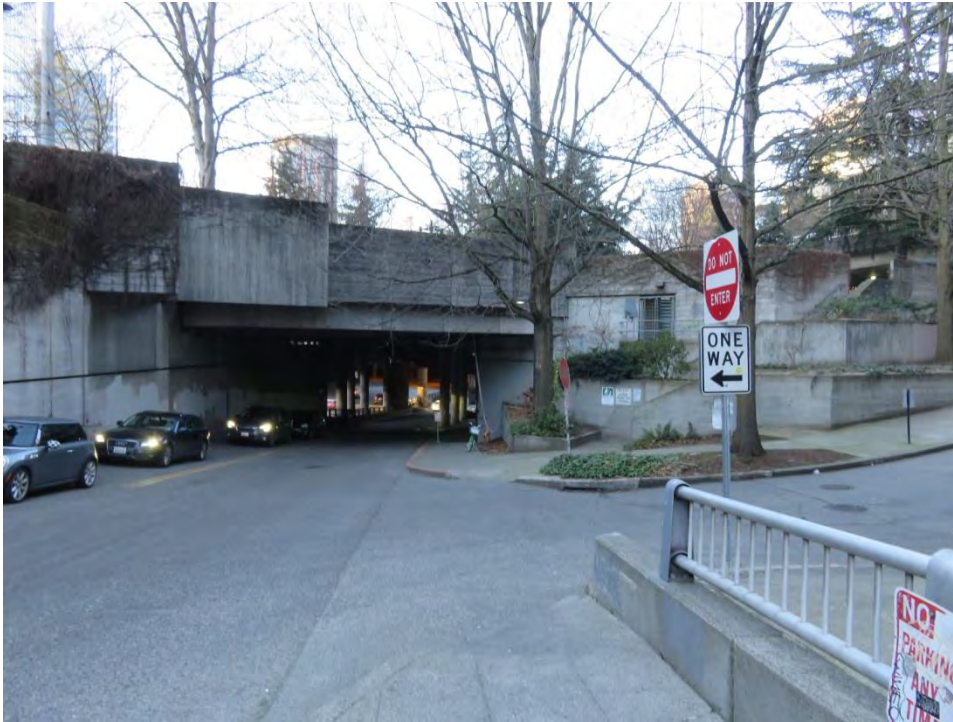
Photo 22 of 28. WA_King County_Freeway Park 0023. Hubbell Pl. as it runs north between I-5 to the west and the Freeway Park Garage to the east, under the Freeway Park lid, view north.
