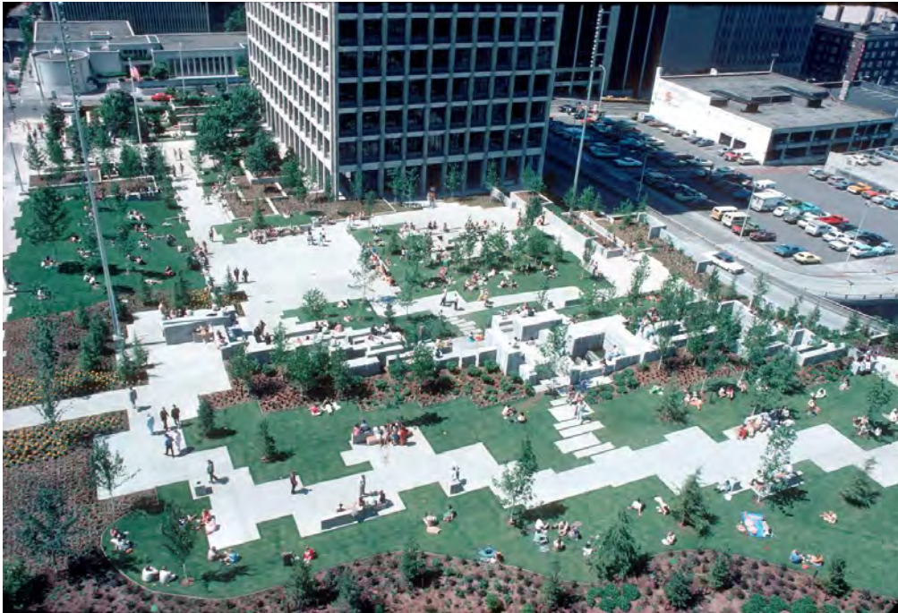
Freeway Park, view to west, July 1976, the month it opened. Image courtesy of Seattle Municipal Archives.
