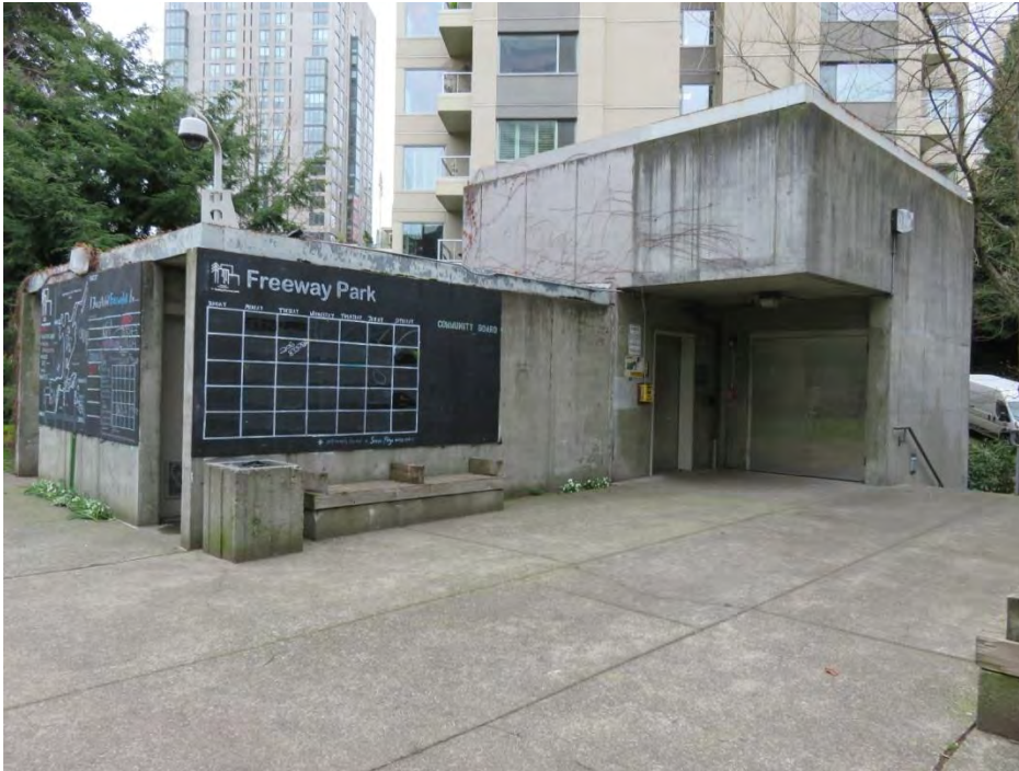
Photo 16 of 28. WA_King County_Freeway Park 0017. Freeway Park Comfort Station and elevator to Freeway Park Garage, view northeast.
