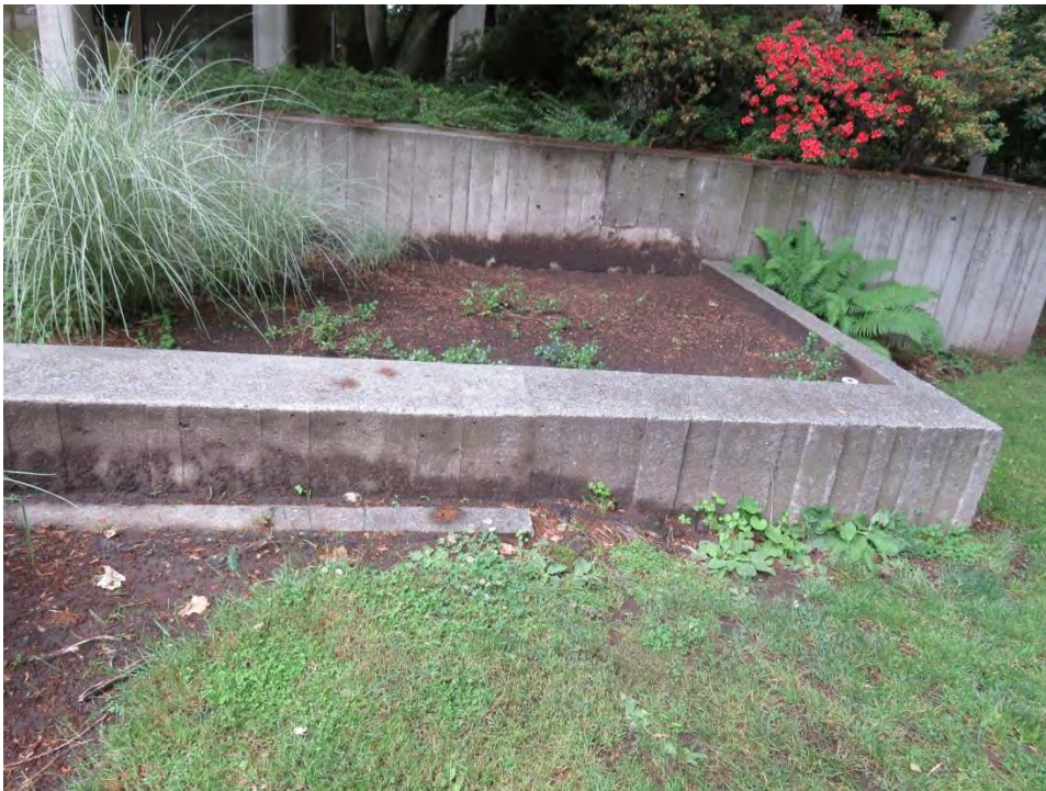
Photo 7 of 28. WA_King County_Freeway Park 0007. The seam, visible in the concrete, between the original Park Place Plaza (ca. 1971) and Freeway Park (1976).
