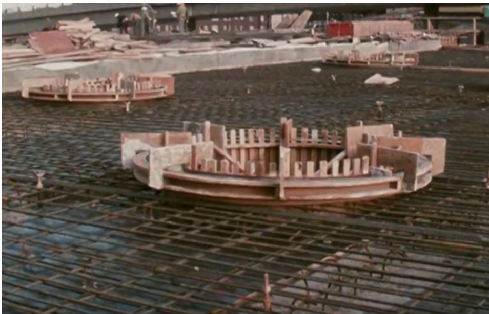
Freeway Park, view showing large tree wells. Image courtesy of Seattle Municipal Archives. Freeway Park and Garage (1st Phase)
