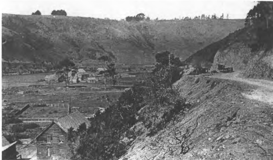
Figure 6. The Inn building view northeast with barns in background, circa 1920. Collection of the Charles Fletcher Society.
