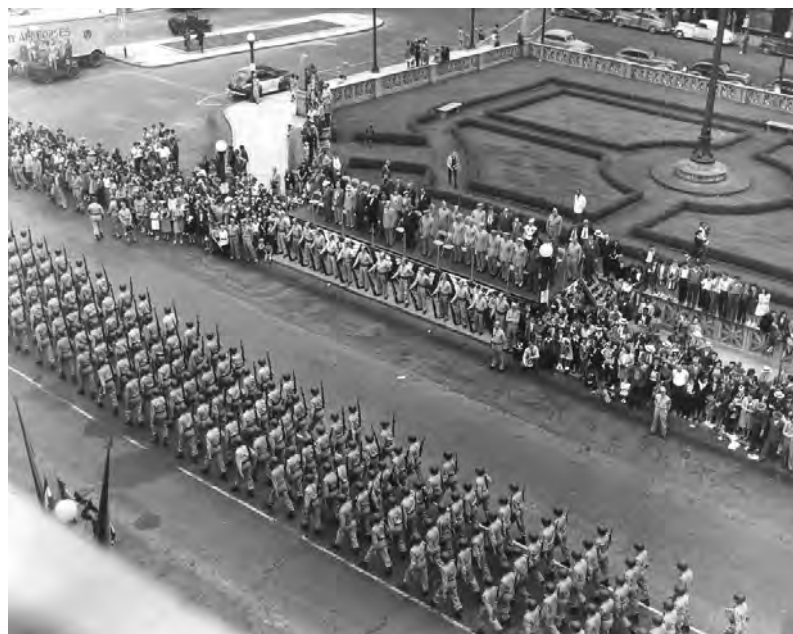
From roof of Tennessee War Memorial, Memorial Day parade, June 3, 1946 RG 82, Box 55, File 60, Image ID 21731
