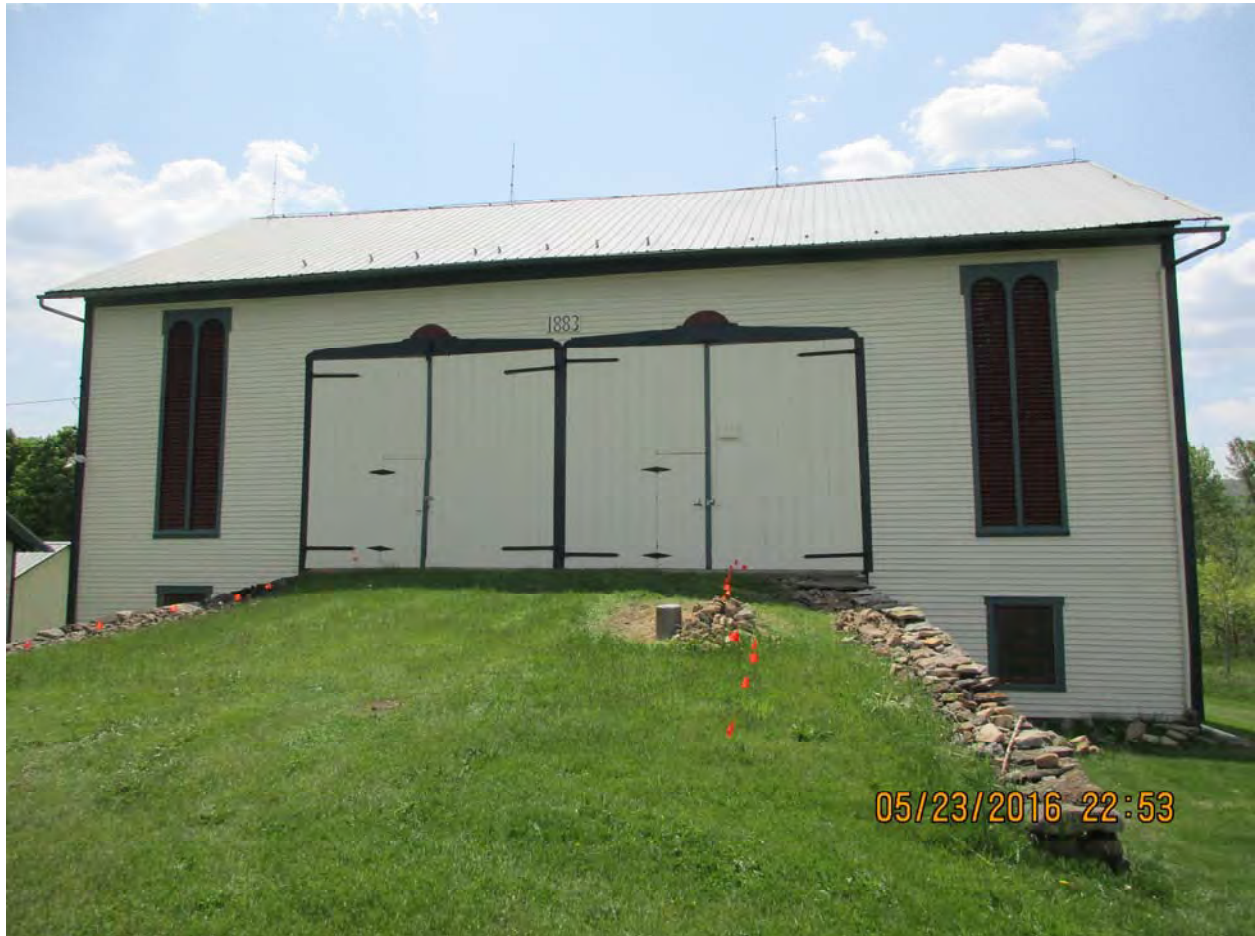
Photo 5: BARN BANK SIDE
