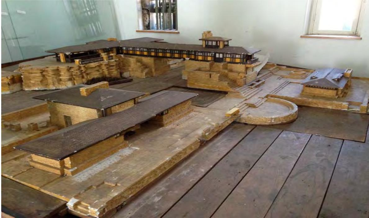
FIGURE 24 Wood and plaster model of Bridge Complex – upper left, Indian Room and restrooms – lower right, patio, and Veranda Rooms on the far right as built. No date for model. Source: Alfred Caldwell drawings, models and plans. City of Dubuque Parks Division, Dubuque, IA.
