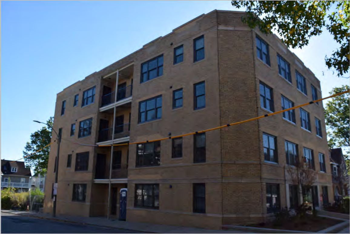
3. Bicknell Street (west) and Bradshaw Street (north) elevations, looking southeast. (October 2017)
