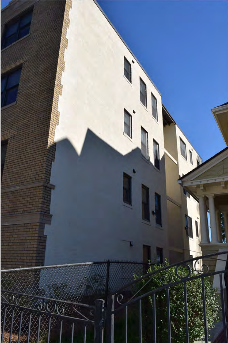
5. South elevation, looking northeast. (October 2017)
