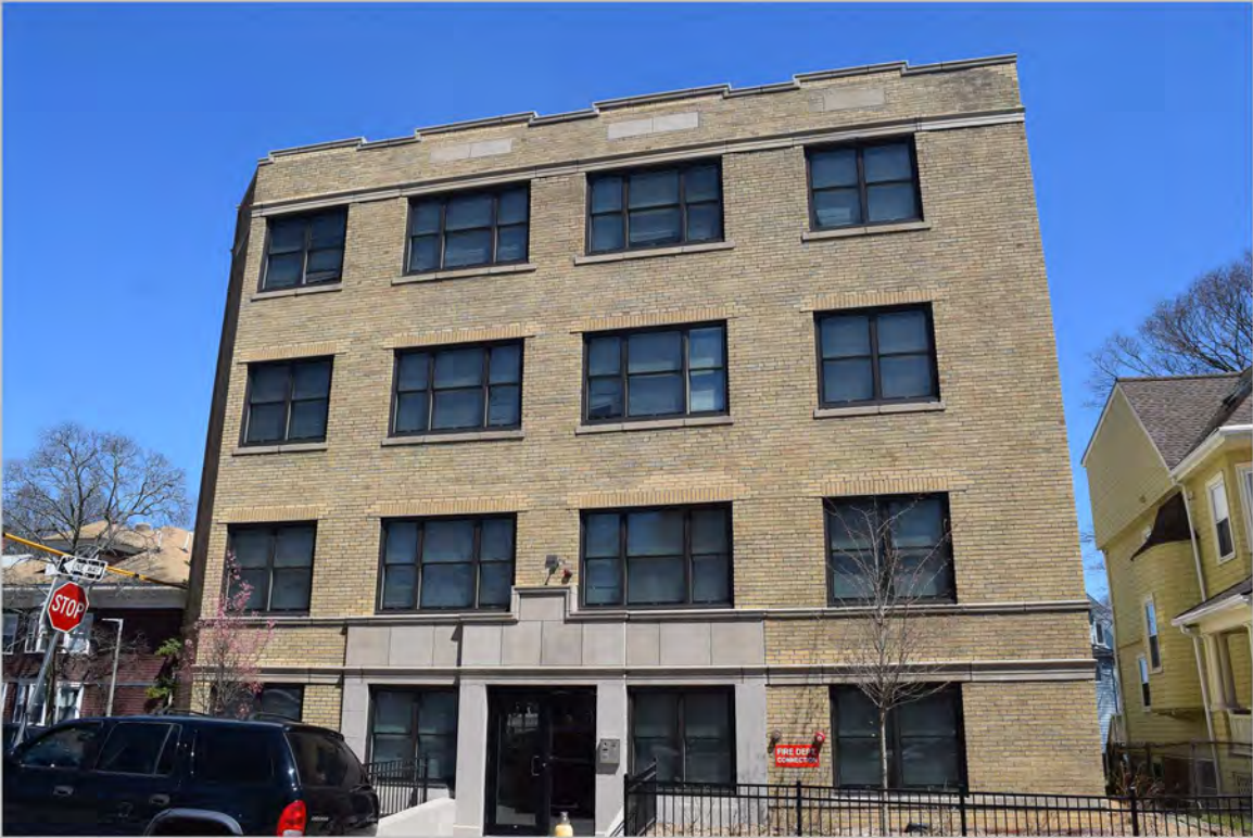
1. Bicknell Street (west) elevation, looking northeast. (April 2017)
