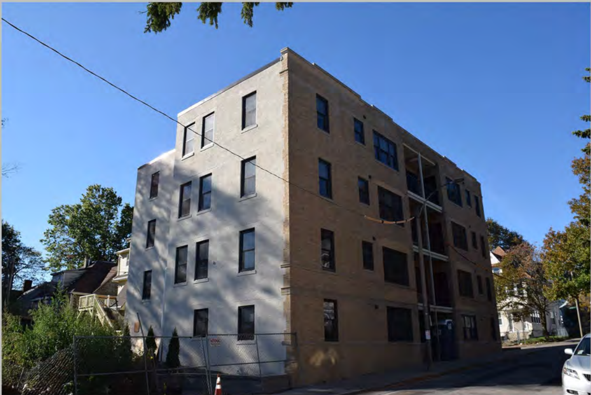
4. East elevation, looking southwest. (October 2017)
