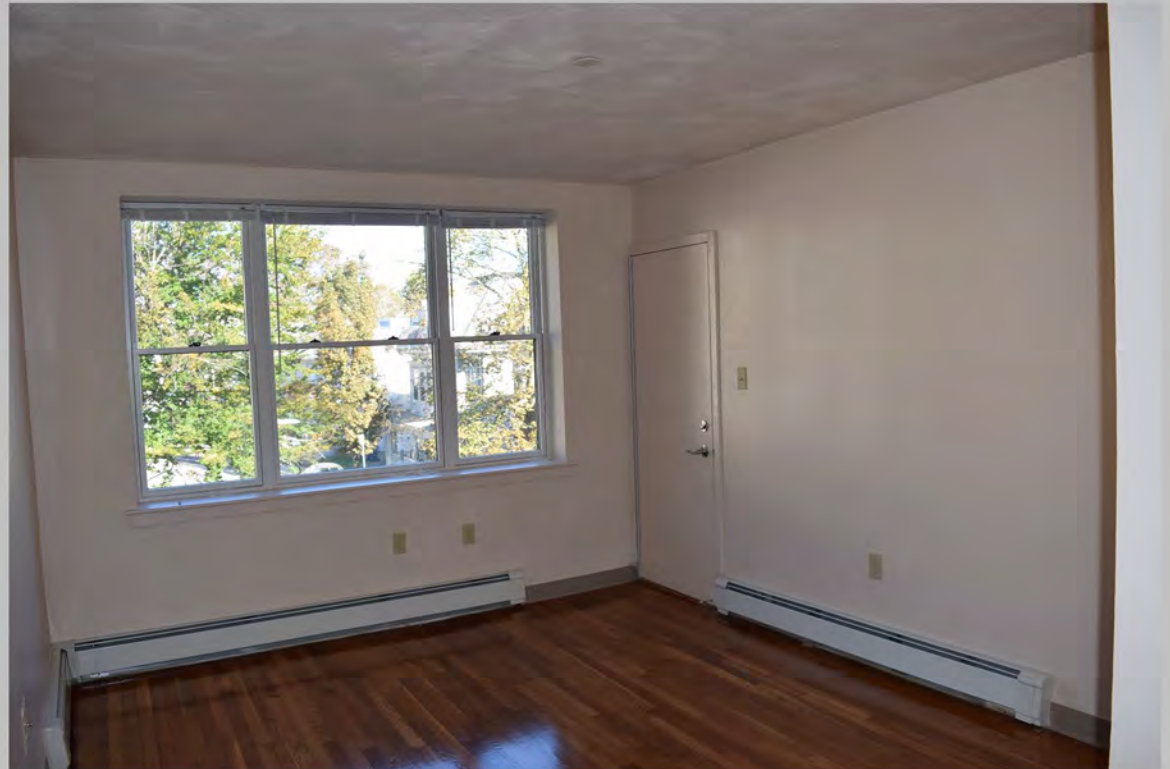
10. Second floor unit living room, looking northeast. (October 2017)
