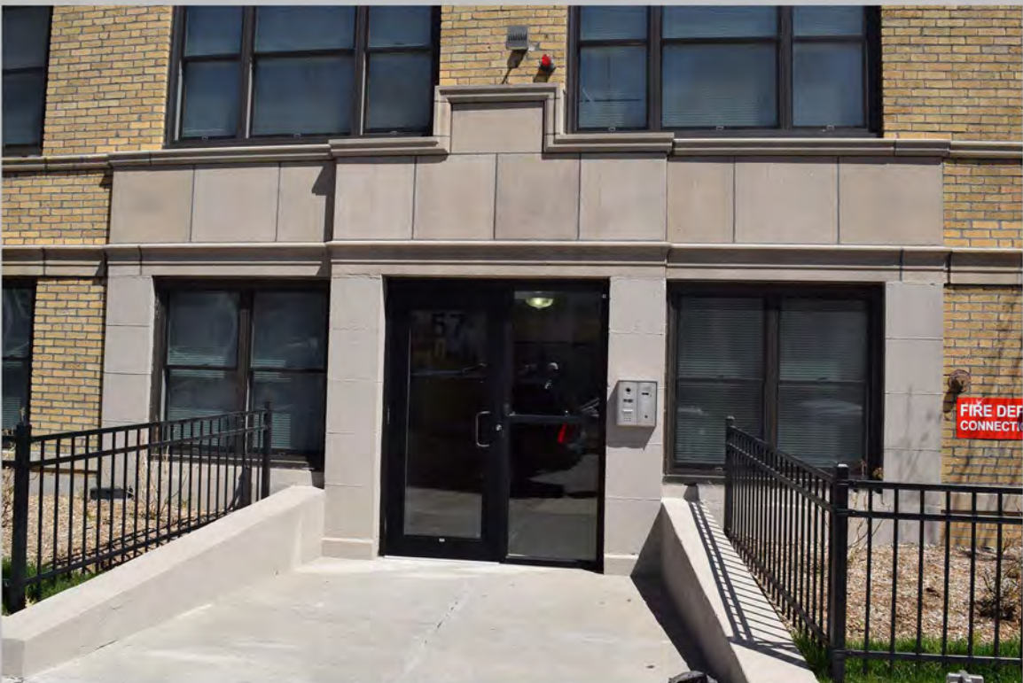
2. Detail of entry on Bicknell Street (west elevation), looking east. (April 2017)
