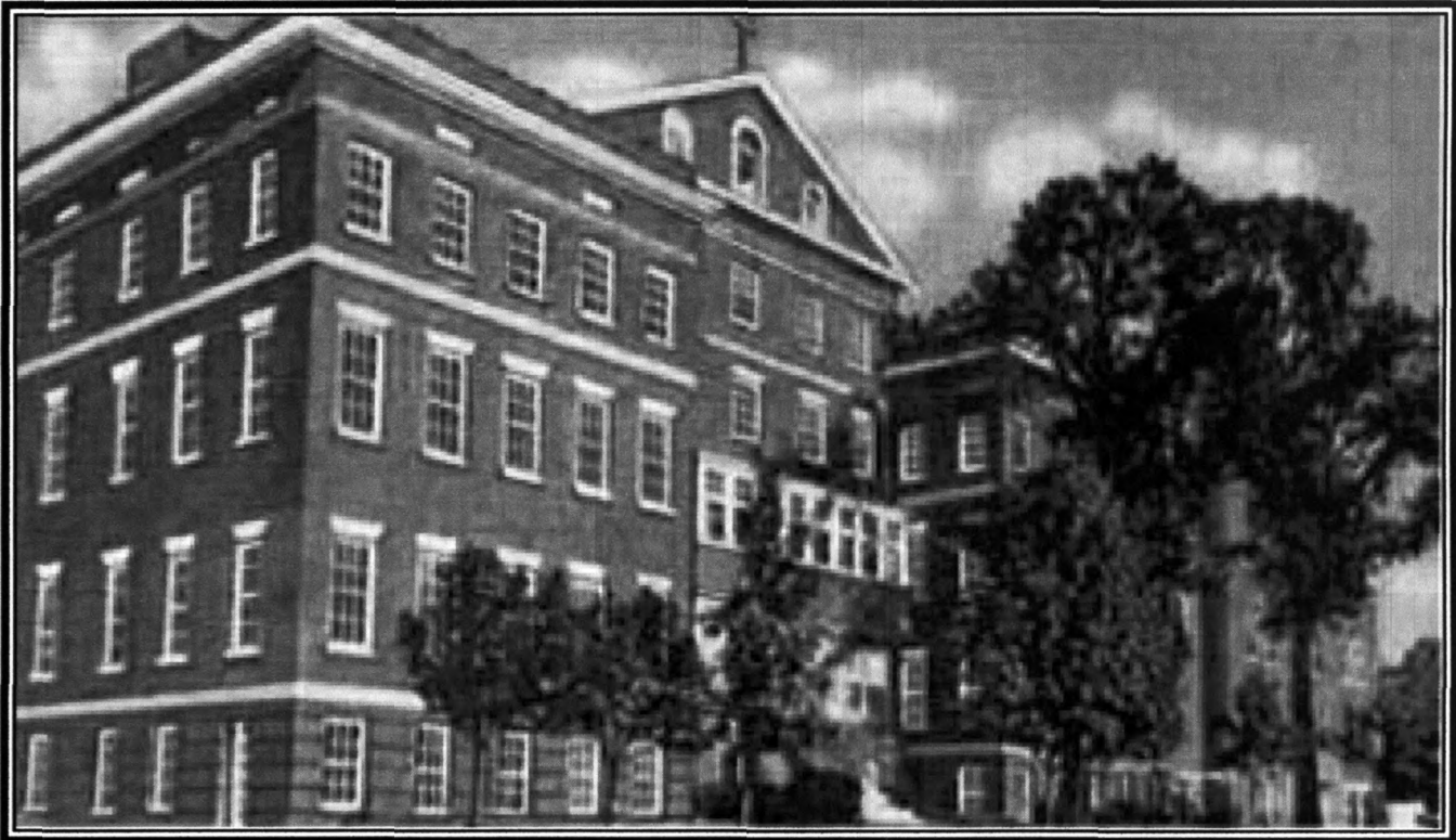
Fig. 1 Sacred Heart Hospital stood on the north side of Decatur Street. Following its demolition, only a stone retaining wall remains; it is an important element in the streetscape of Decatur Street and is a tangible reminder of the presence of the hospital in the neighborhood for decades.
