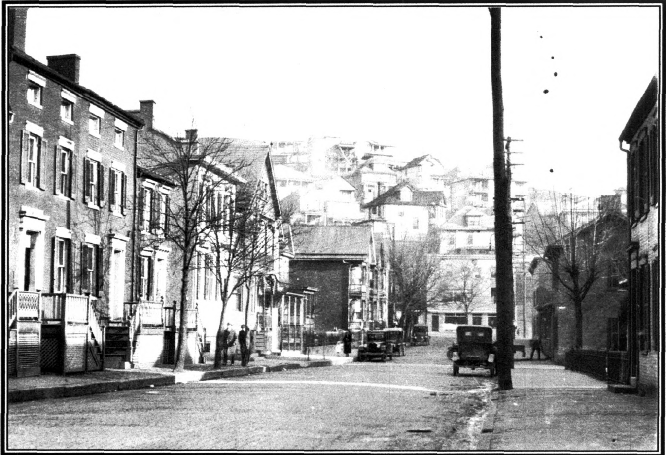
Fig. 2 This 1920s [photo shows the Federal-Greek Revival architectural character of Decatur Street, much of which has been retained. This view is looking eastward toward the steep hillside along Baltimore Avenue. [City of Cumberland, Herman and Stacia Miller Collection]
