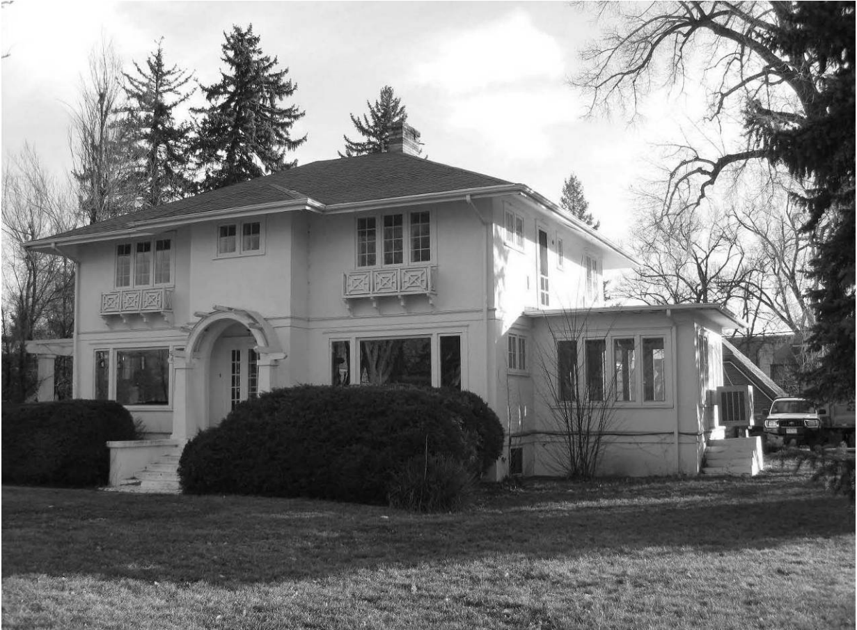
Figure 7: Prior to rehabilitation, 2014. On file with preparer.
