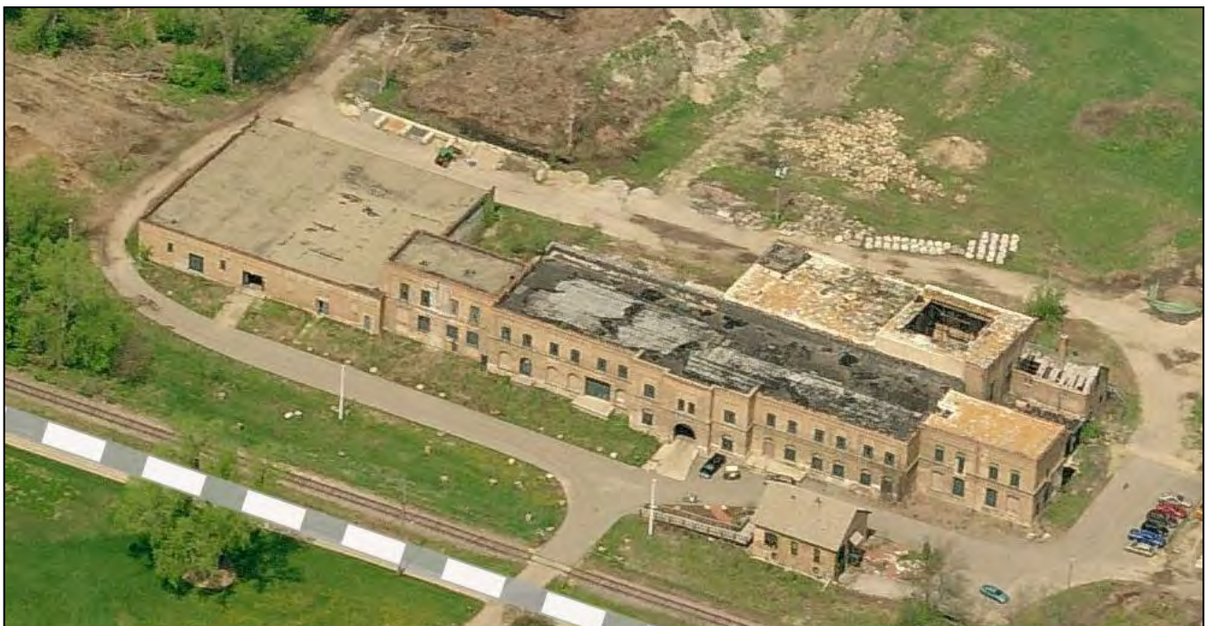
Figure 5: Aerial view of Garver's Supply Company Factory and Office, looking north
