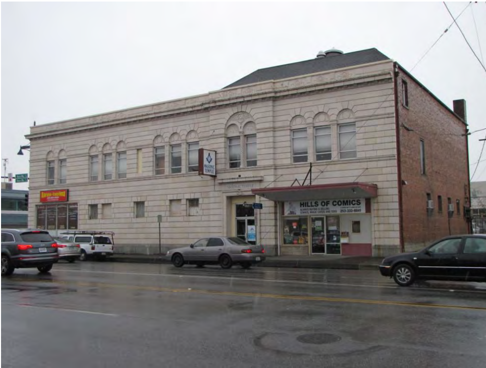
2 of 13 West façade facing Auburn Way.
