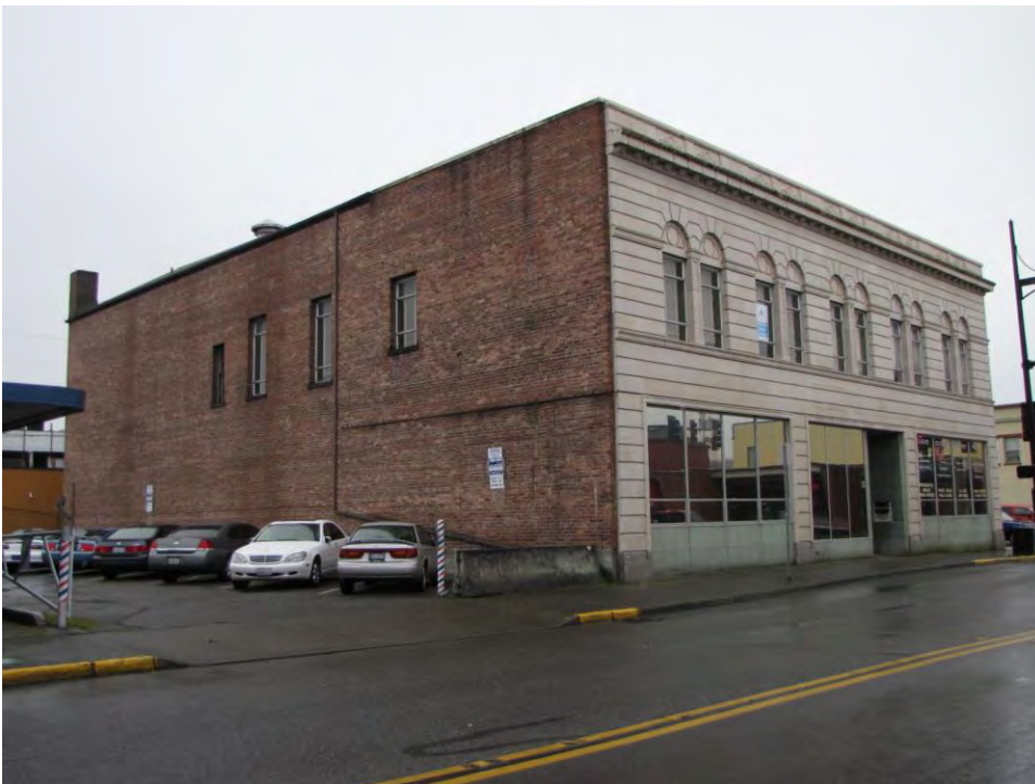
3 of 13 Northeast corner looking south showing side façade facing parking area.
