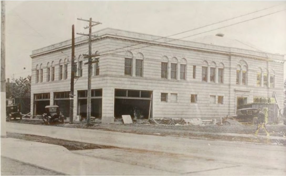
Photograph of nearly completed Temple building.
