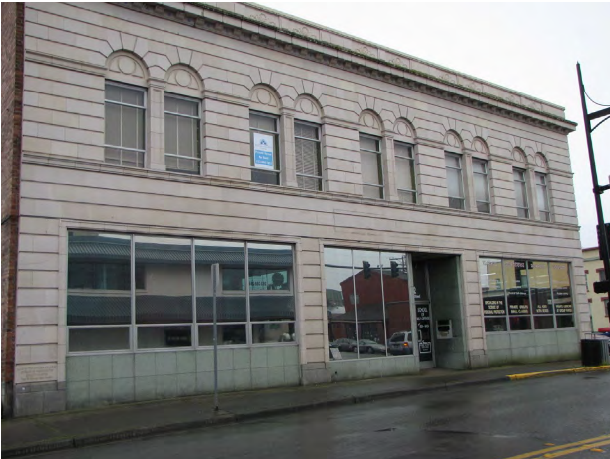
1 of 13 North façade facing E. Main Street.
