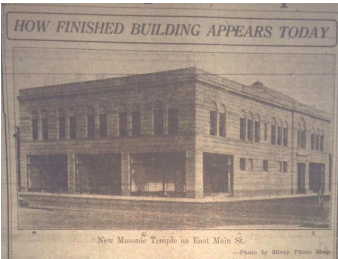
Photograph of nearly completed Temple building – Auburn Globe Republican , August 1, 1924.
