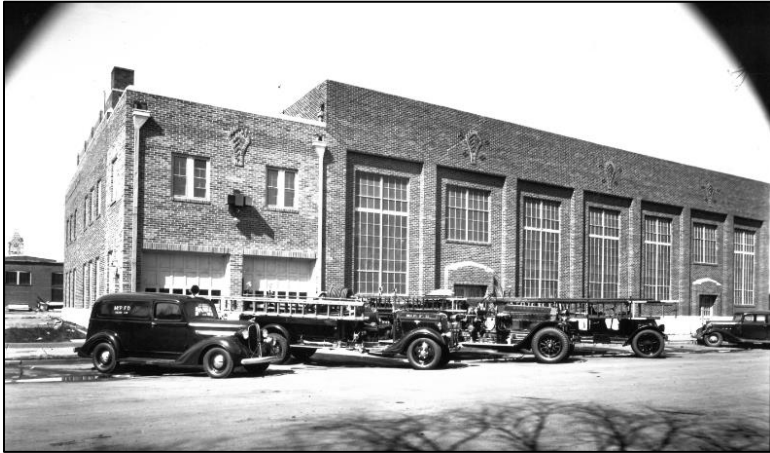
Figure 11: East elevation shortly after 1934 when the fire station expanded.
