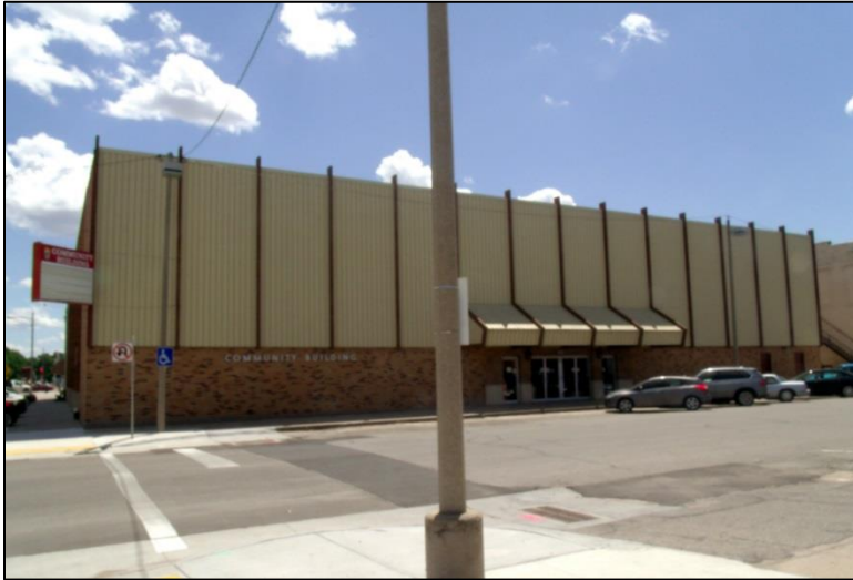
Figure 12: The north façade of the McPherson Community Building as it appears in early 2017 before the historic façade was revealed by the removal of the 1970s addition.
