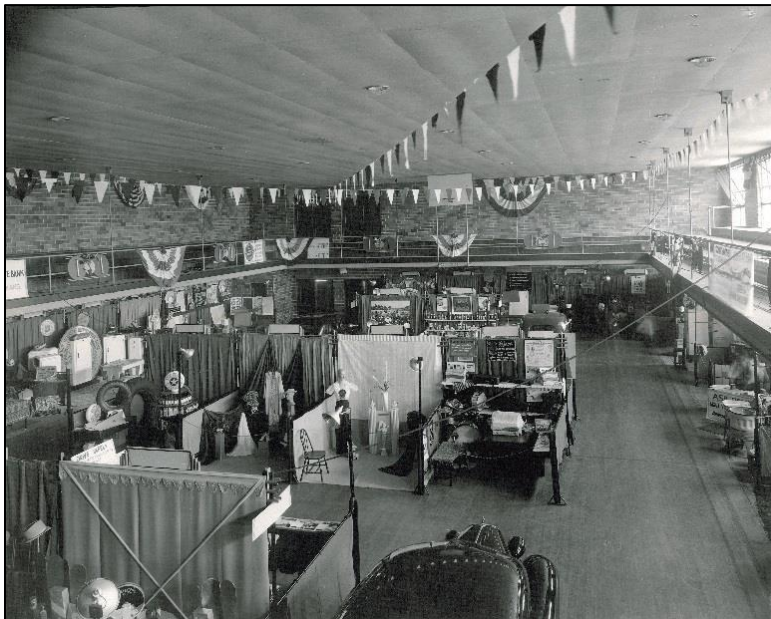
Figure 6: Gymnasium, looking north from the south mezzanine, showing the finished historic ceiling at an unknown date.
