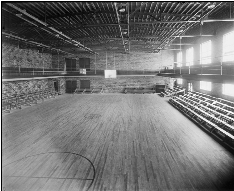
Figure 7: Gymnasium shortly after construction, looking north and showing exposed ceiling.
