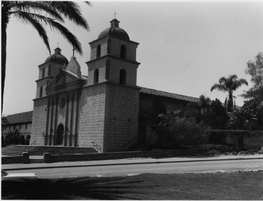
Santa Barbara Mission Church, 1815-20 East (front) and north (side) elevations
