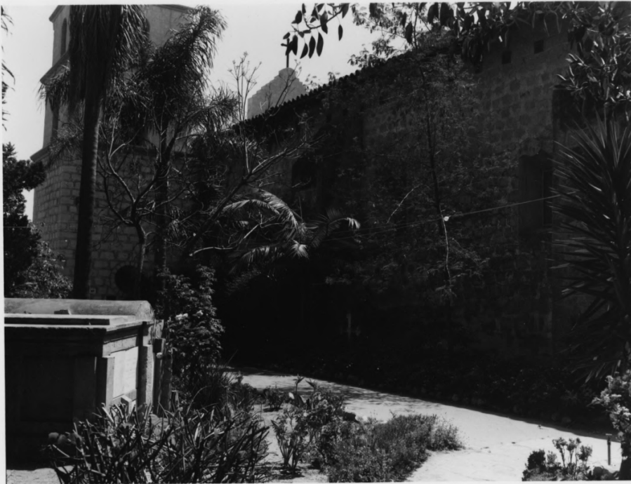
Santa Barbara Mission Church, 1815-20 East (side) elevation 2201 Laguna Street Santa Barbara, California
