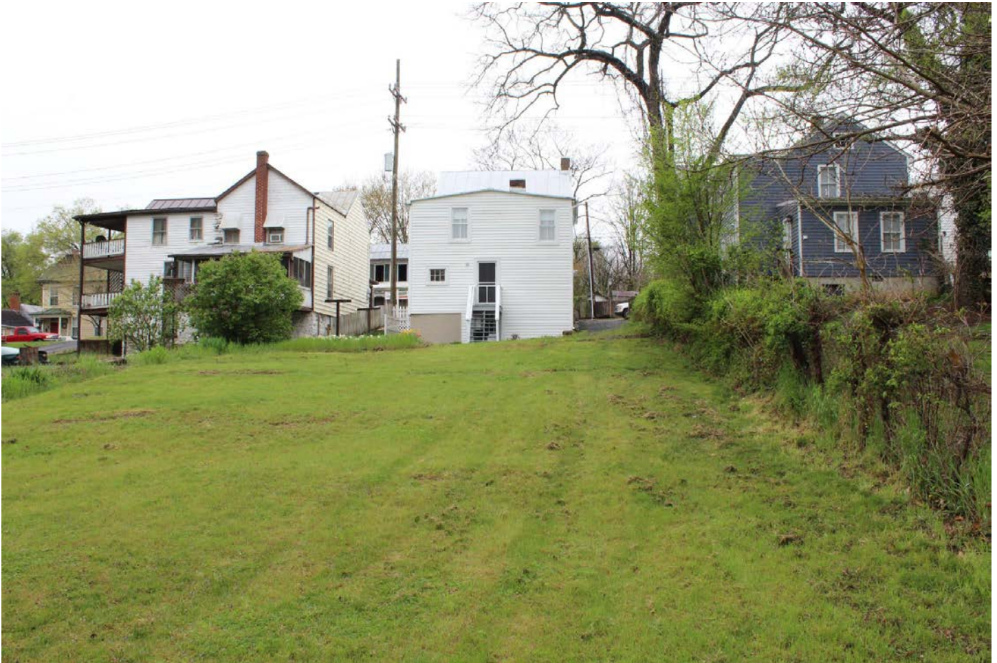
Photo 5. Exterior, looking west, showing backyard and east elevation. April 2018.
